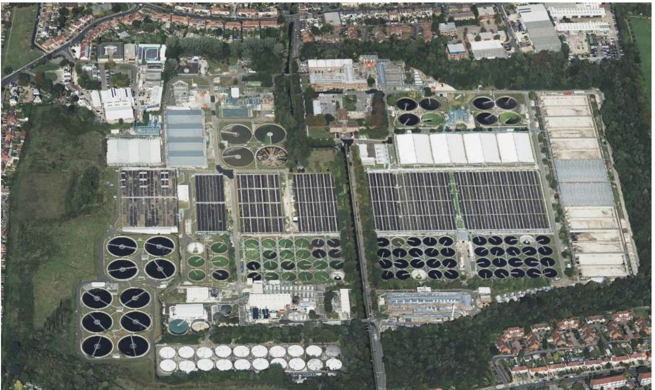
Figure 2-1 - Satellite view of Mogden Sewage Treatment Works
