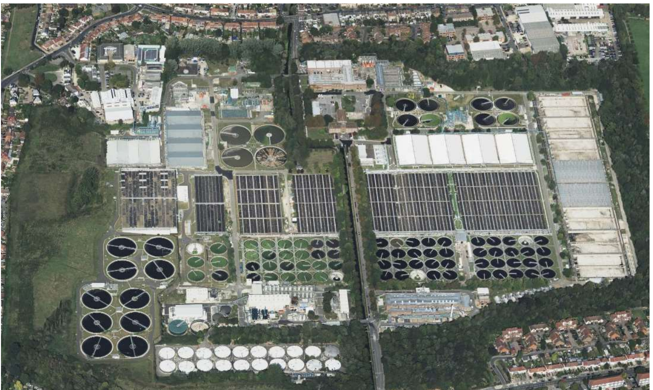
Figure 2-1 - Satellite view of Mogden Sewage Treatment Works
