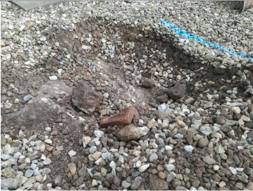
Figure 2: View of Trial Pit 1
