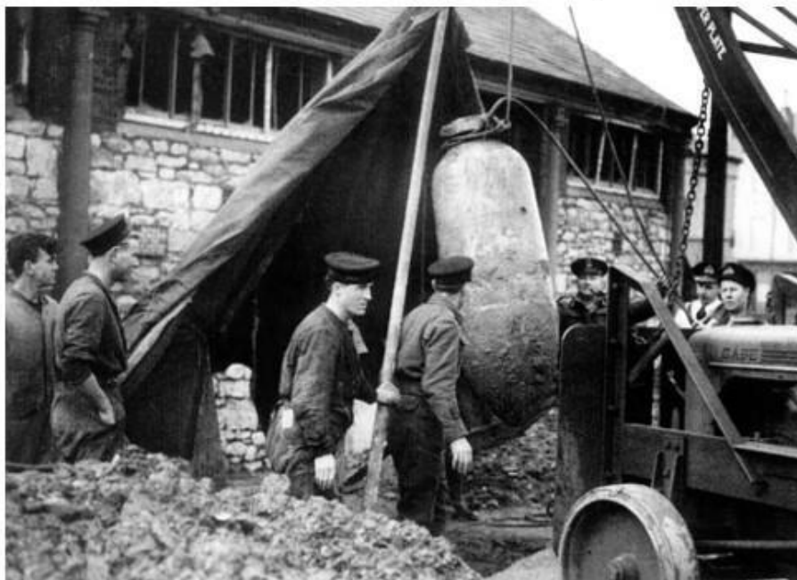
Removal of an UXB
