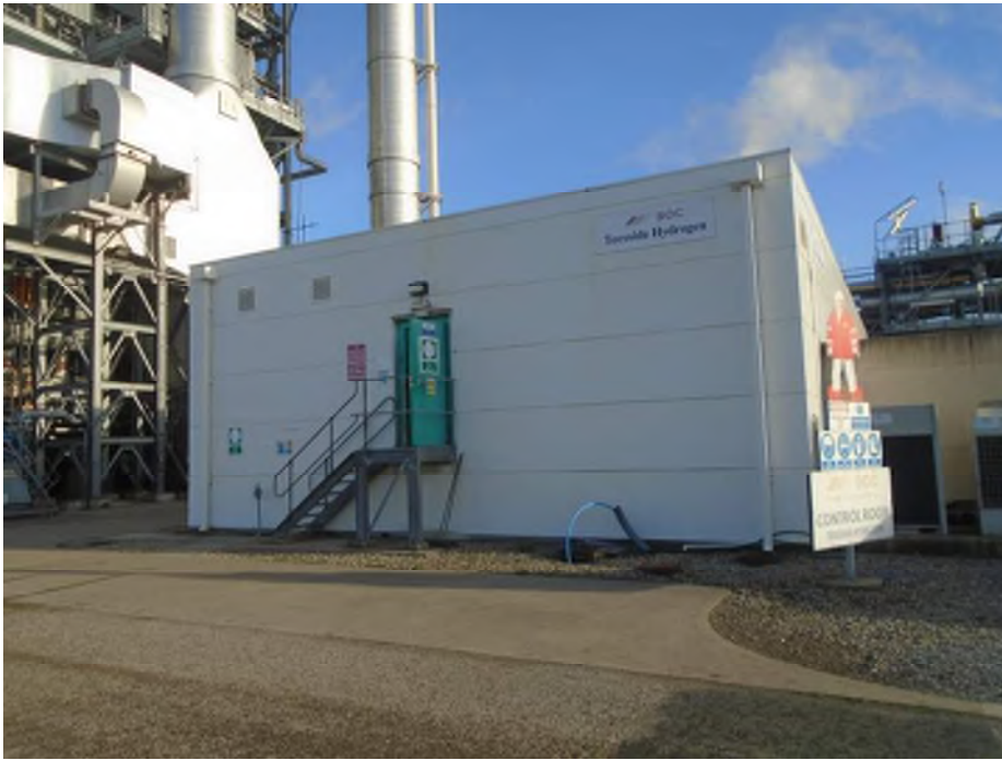
Photograph 1: General view of Site – control room & offices.
