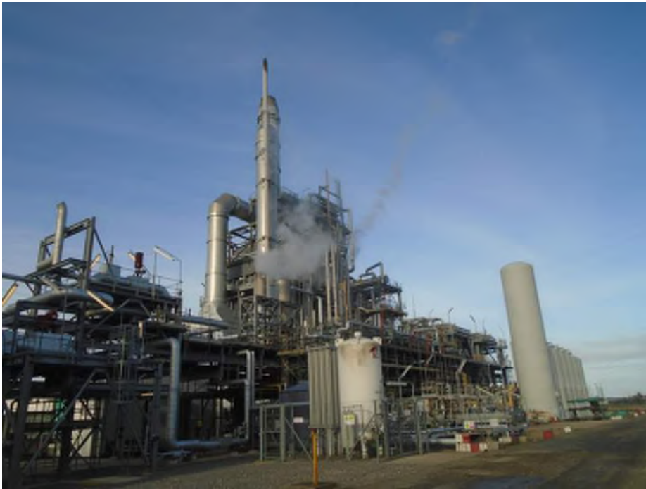
Photograph 3: General view of Site – viewing northeast towards the hydrogen plant.
