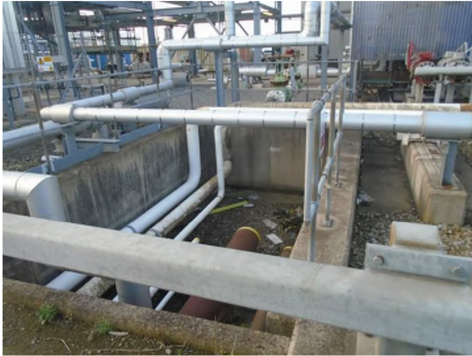
Photograph 5: Culvert off-site to the west (raw natural gas feed inlet, end-product hydrogen feed to clients and effluent feed to SABIC treatment facility).
