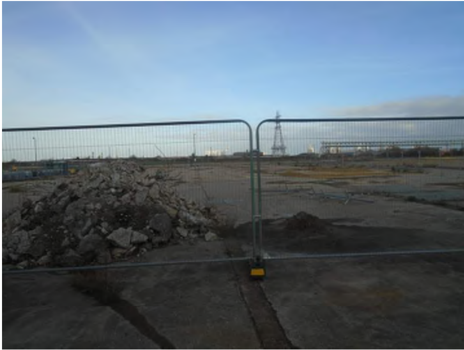
Photograph 22: General view of the northern area of the Site intended for development (expansion of the existing hydrogen plant).
