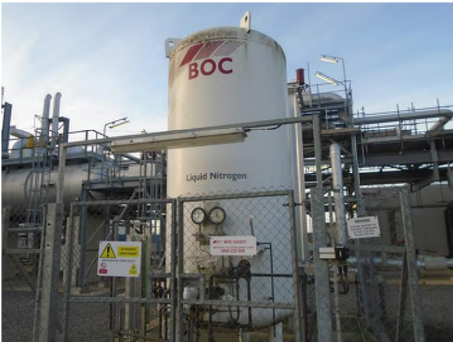
Photograph 4: 2080L liquid nitrogen above ground storage tank (AST) located in the west of the Site.
