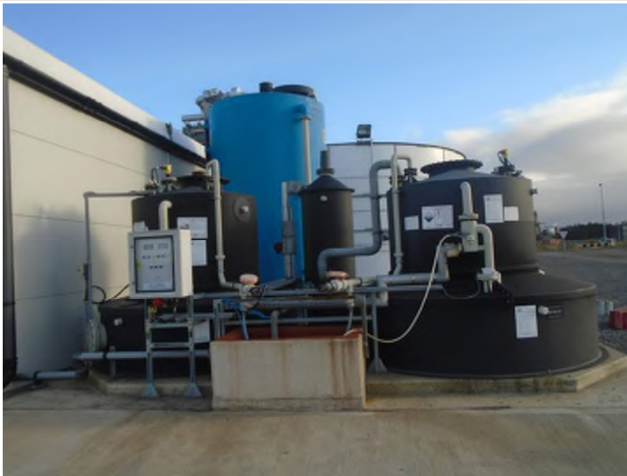
Photograph 21: Internally banded ASTs containing chemicals for water treatment (Caustic Soda Liquor and Hydrochloric Acid, 3000L and 4000L capacity respectively).
