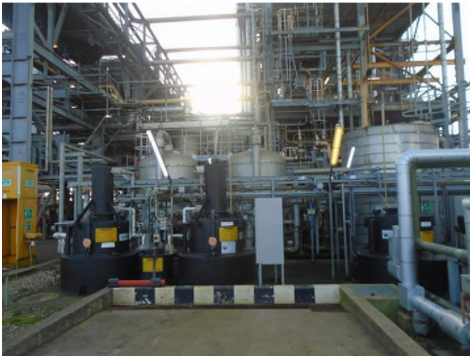
Photograph 8: Internally banded ASTs containing chemicals for water treatment (Ammonia, HCL, Drewphos, Amersite, Sulphuric Acid and Sodium Hypochlorite, 1500L to 2500L capacity).
