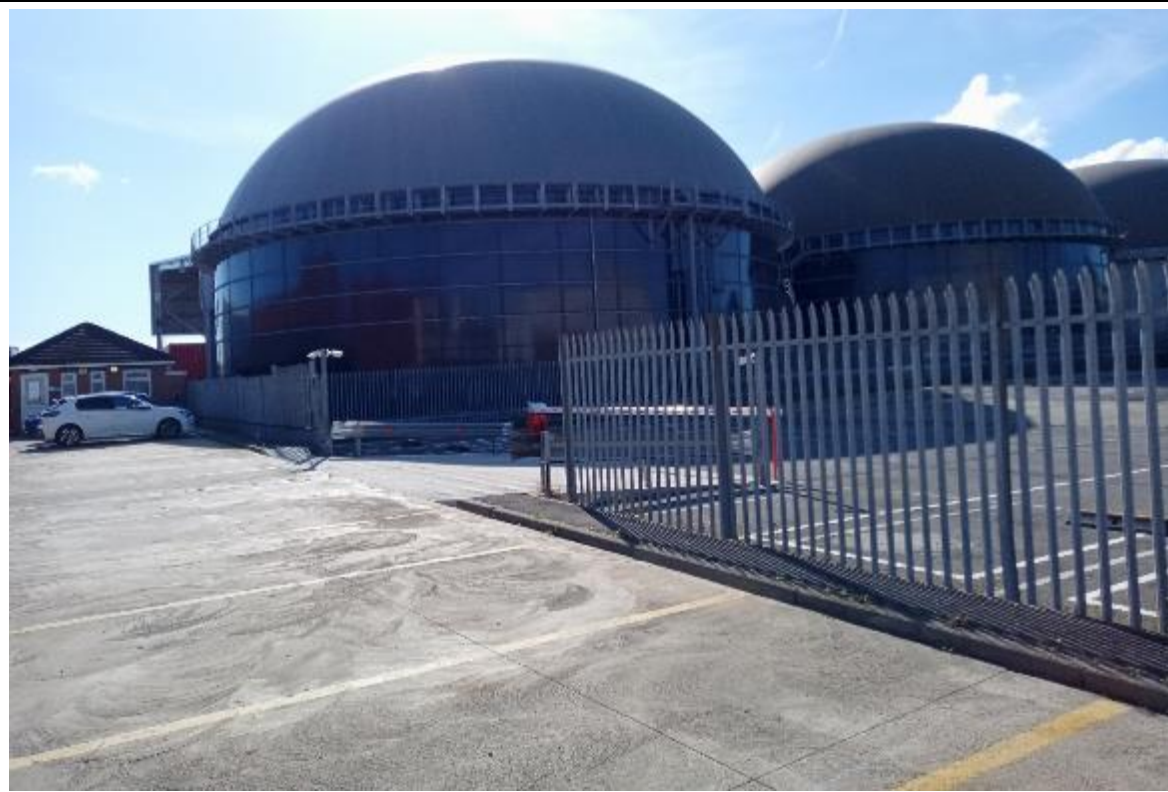
Photo taken offsite to the north, looking east towards the Duranta digestate storage tanks. The vehicle access point to the site on the northern boundary is shown.
