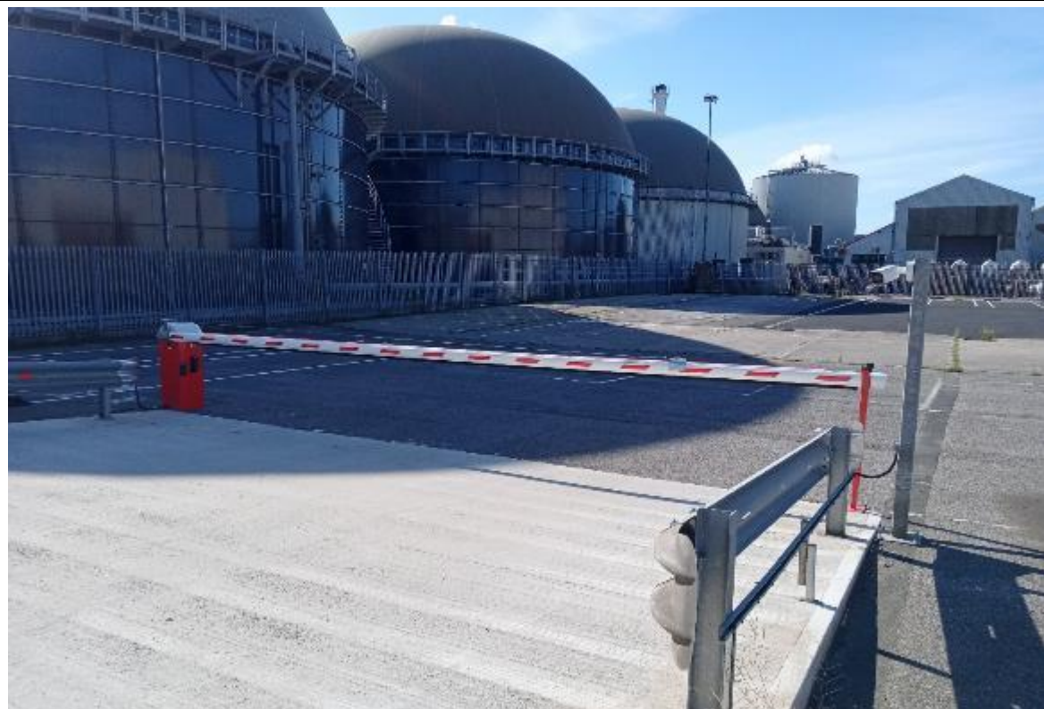
Photo looking south at the site from the vehicle entrance point. The site comprises the asphalt surface lorry park. Propane storage tanks and buildings beyond are offsite to the south of site. The digestate storage tanks are offsite to the east.
