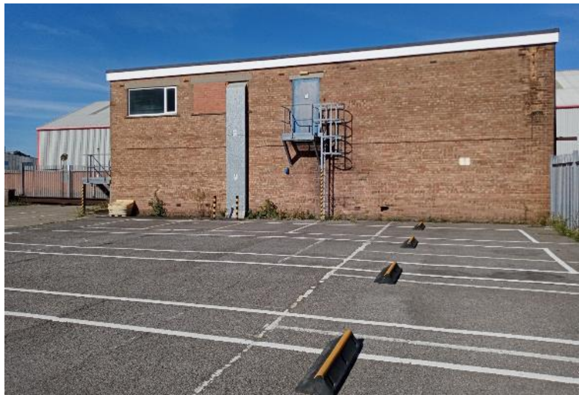
Photo looking west in the north of the site. An electrical substation was present in the northeast corner of the site within a secure masonry building. The surrounding ground was surfaced with asphalt and used as a lorry park.
