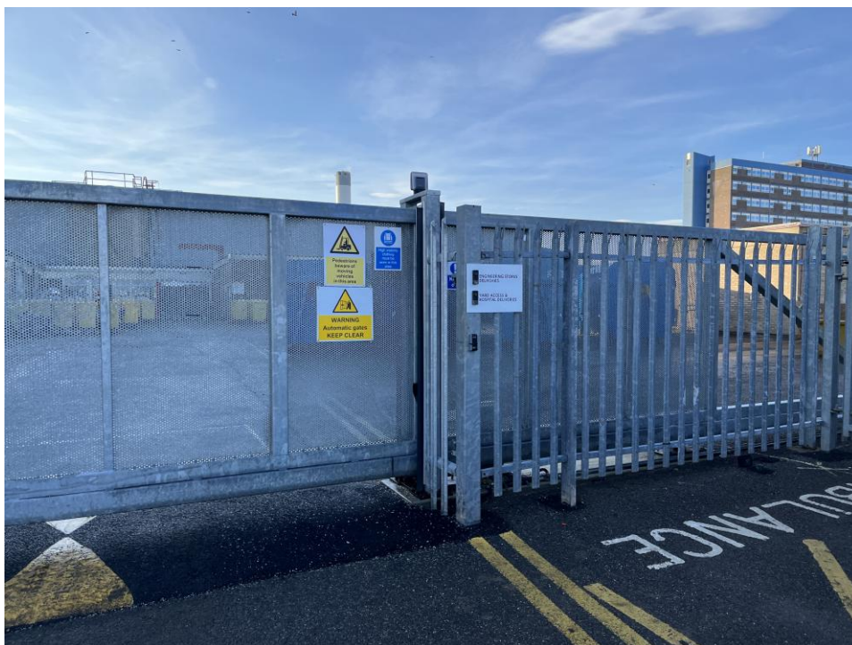
Image 6 Site Entrance/Exit gates
