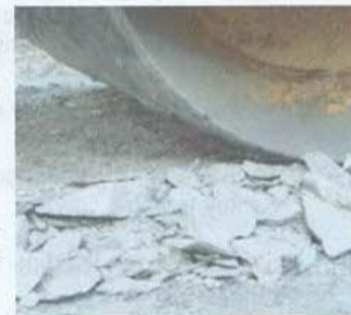
The photo shows large shale pieces pulverised by 4 passes of a heavy vibrating roller
