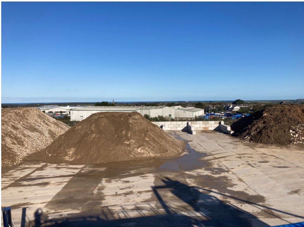
Photograph 10: General view of Site, looking in a northerly direction. Photograph by Horizon, 11 October 2024
