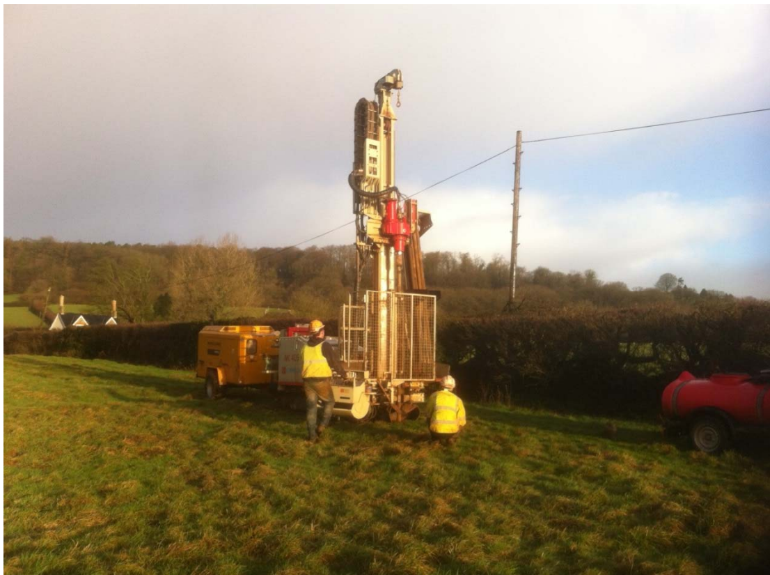
Drilling to prove limestone at Alston - Jan 2015
