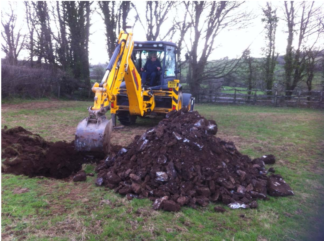
Above: JCB excavating Trial Pit N0.1. Below: Bedding exposed in Trial Pit No.1.
