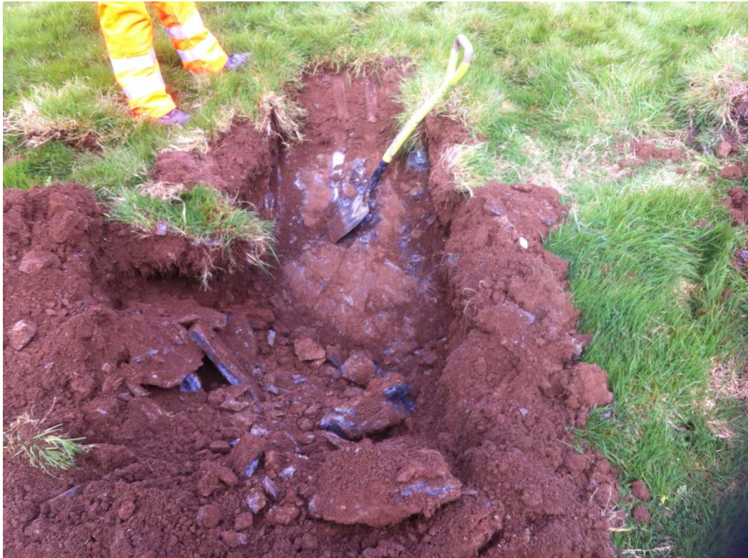
Above: Trial Pit 2 – Bedding exposed in pit. Below: Bedding exposed on A38 roadside, east of planned extension
