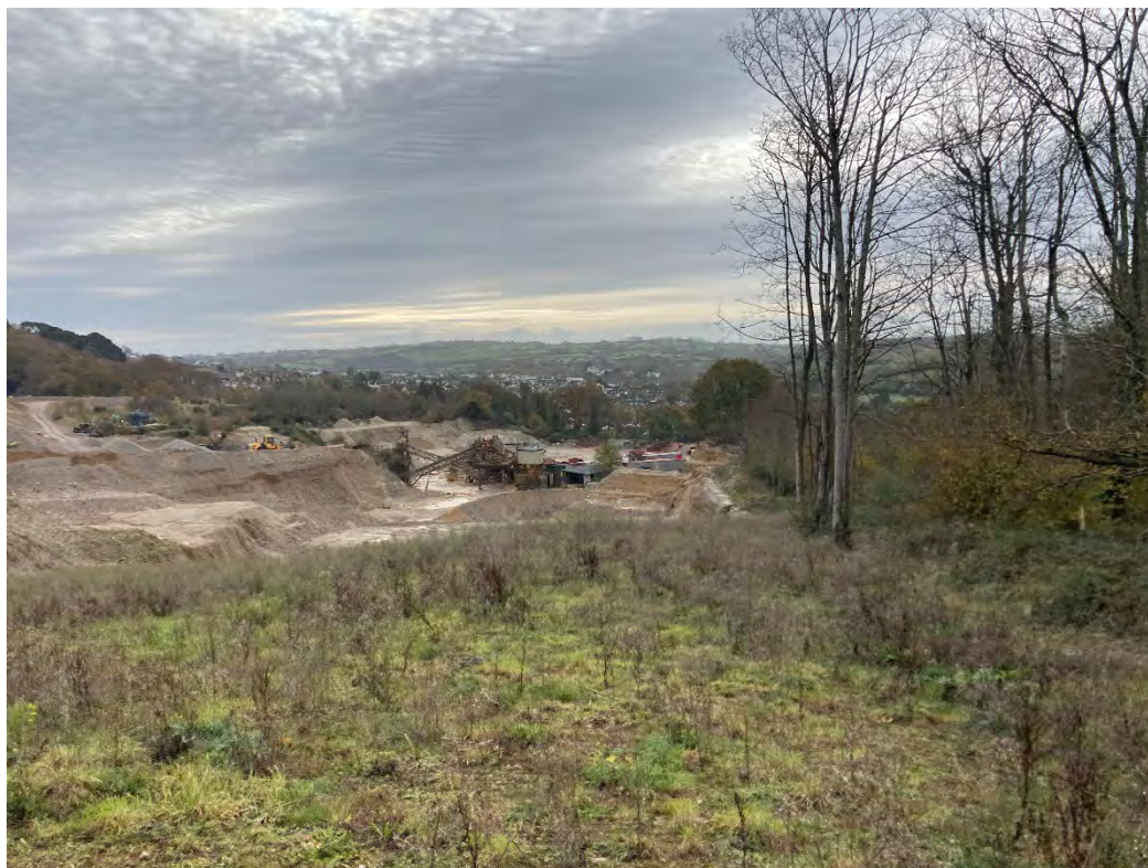
Photograph 07: View along northern boundary of Site, looking in a south-south-westerly direction. [17 November 2023].
