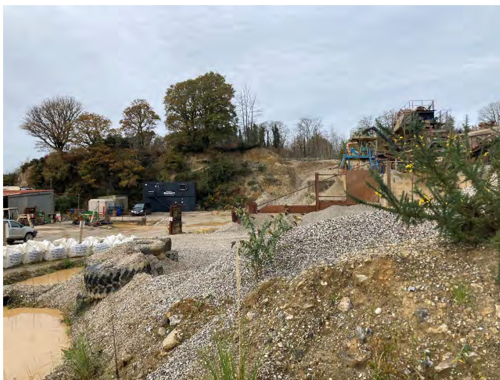
Photograph 06: Working platform and processing plant with exposed slopes (northern boundary) beyond. Looking in a northerly direction. [17 November 2023].
