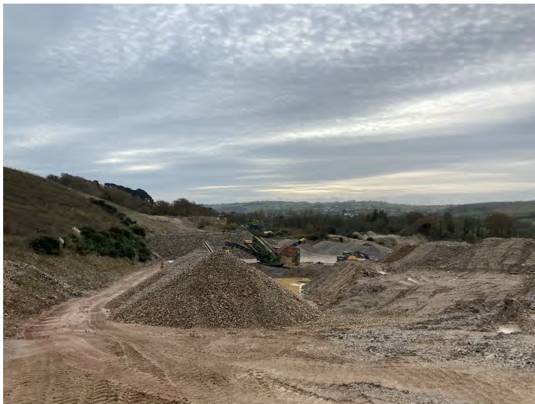
Photograph 03: View of processing plant and working platform in centre of Site, looking in a southerly direction. [17 November 2023]
