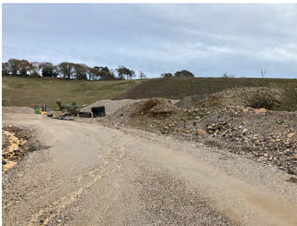
Photograph 04: View of top (north-east) of working platform with eastern slopes in background. Slopes have been partially restored under existing Environmental Permit. [17 November 2023]
