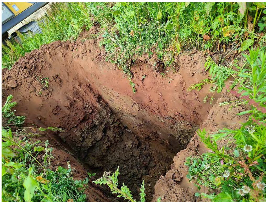
Photograph 5: View of trial pit HTP03.
