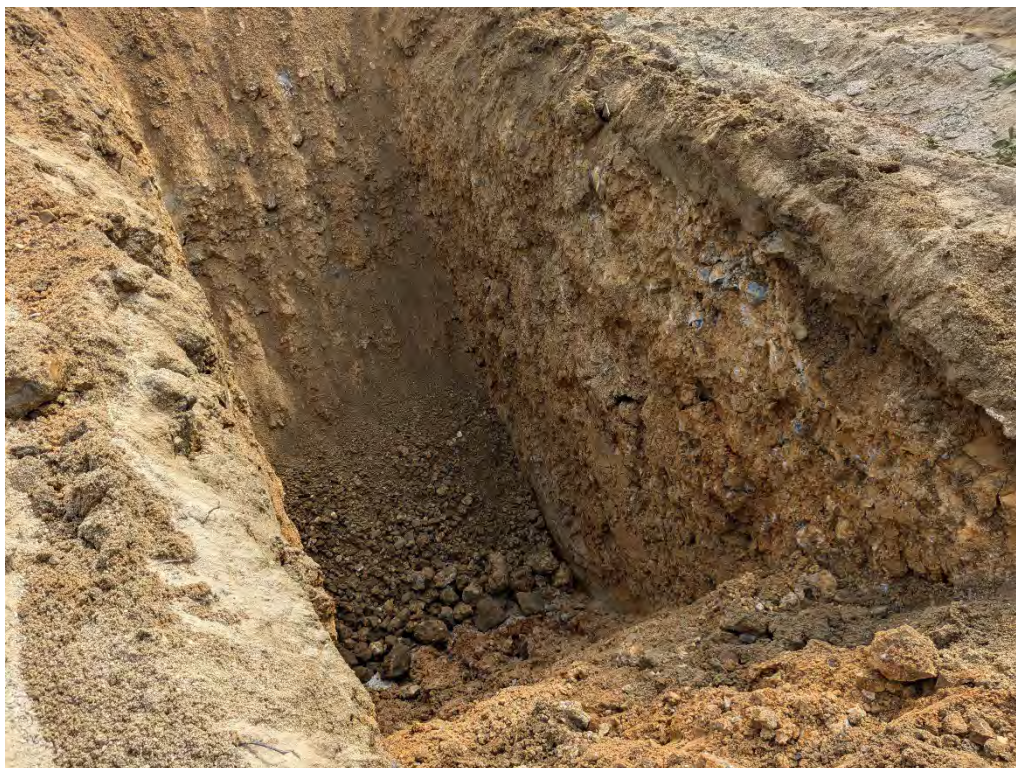
Photograph 9: View of trial pit HTP05.
