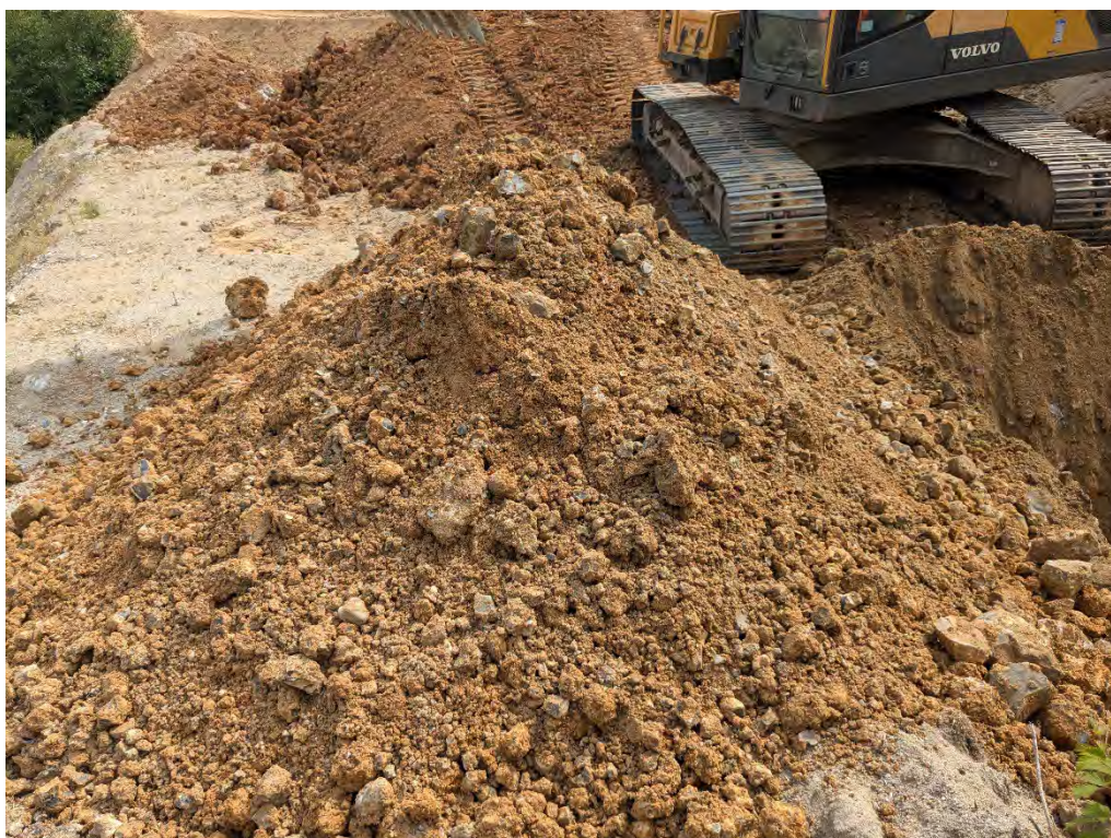
Photograph 10: View of arisings from trial pit HTP05.
