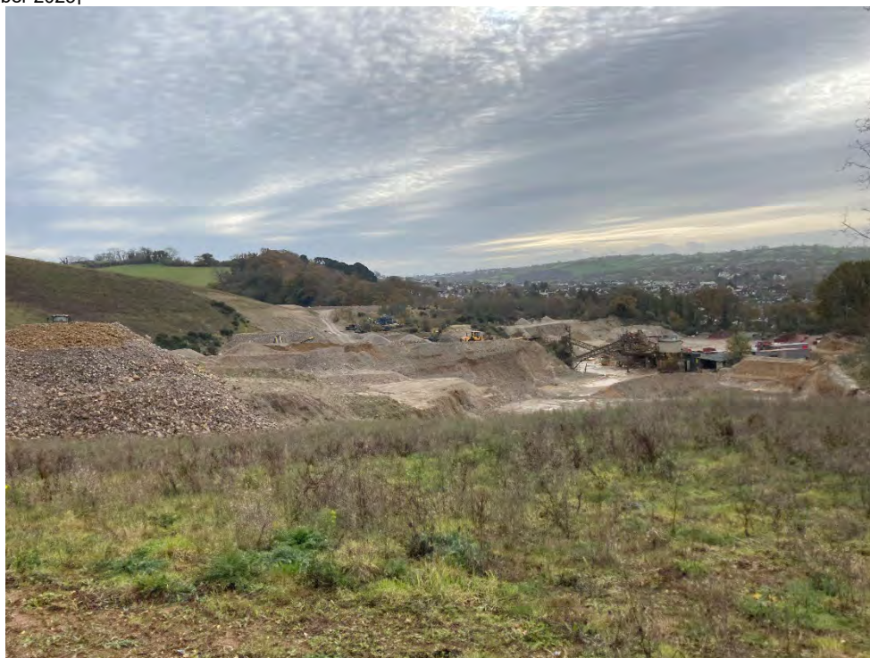
Photograph 02: View of processing plant and working platform in centre of Site, looking in a southerly direction. [17 November 2023]
