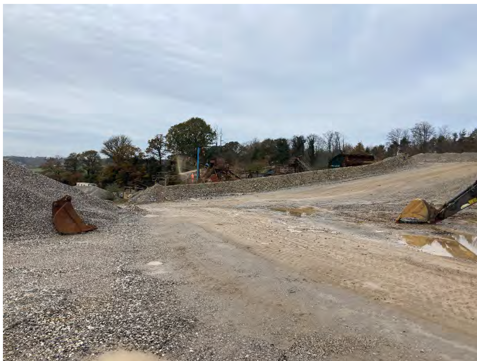
Photograph 14: View of working platform and processing plant, looking in a north-westerly direction. Material still to be extracted in front of photo. [17 November 2023].
