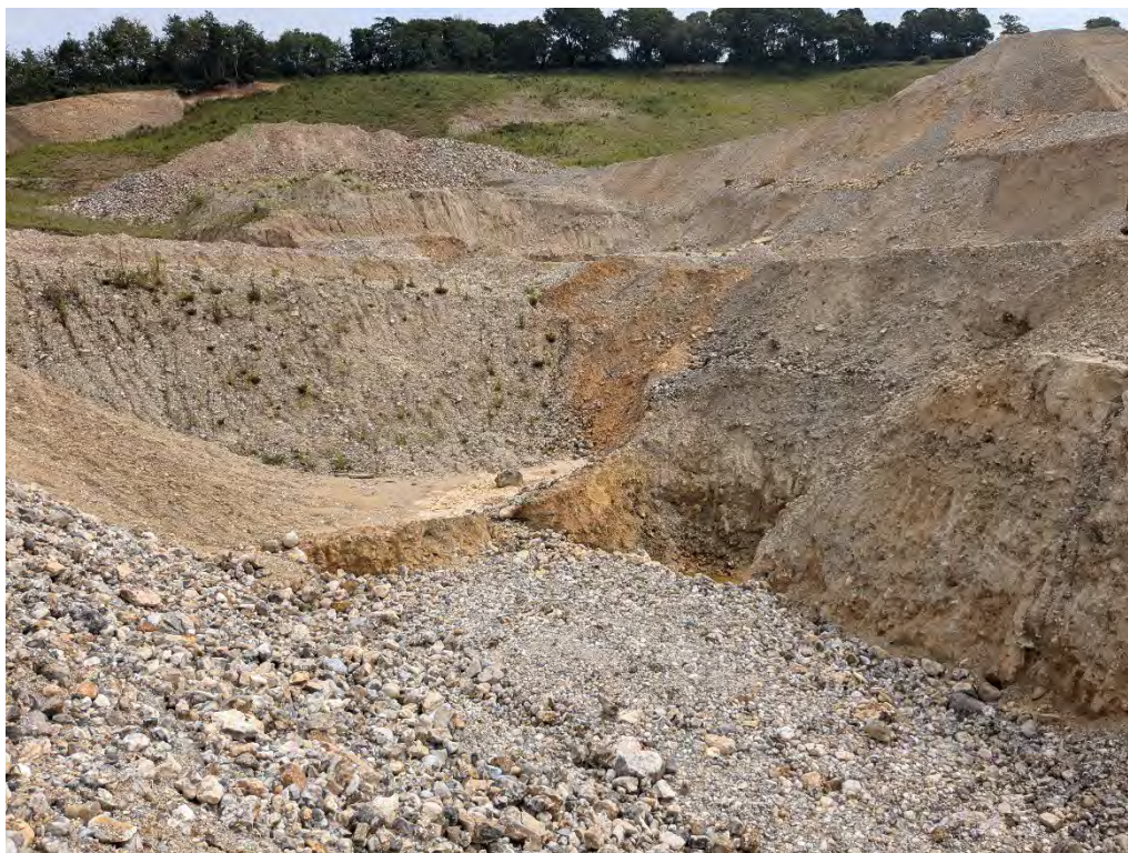
Photograph 13: View of stepped excavations into natural geology in the north-west of the Site.
