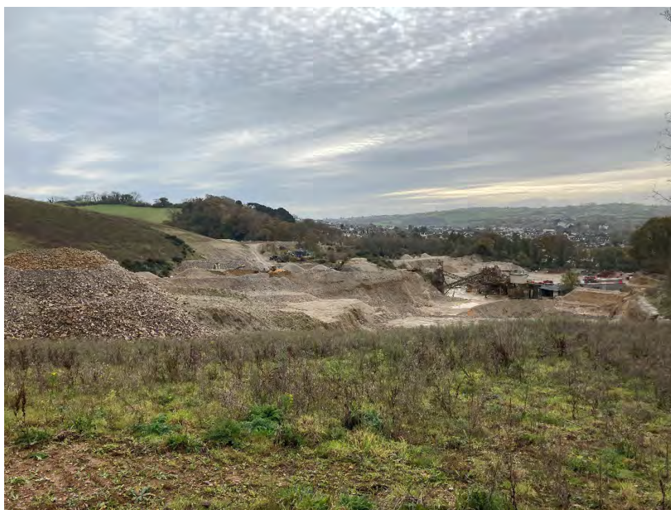
Photograph 08: View working platform looking in a south-easterly direction. [17 November 2023].
