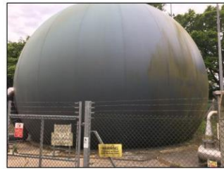
Figure 9: Double membrane gas bag.
