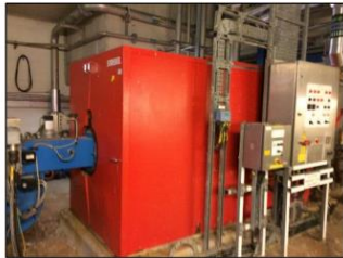
Figure 7: Gas boiler
