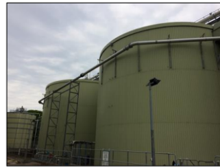
Figure 3: Sludge digesters
