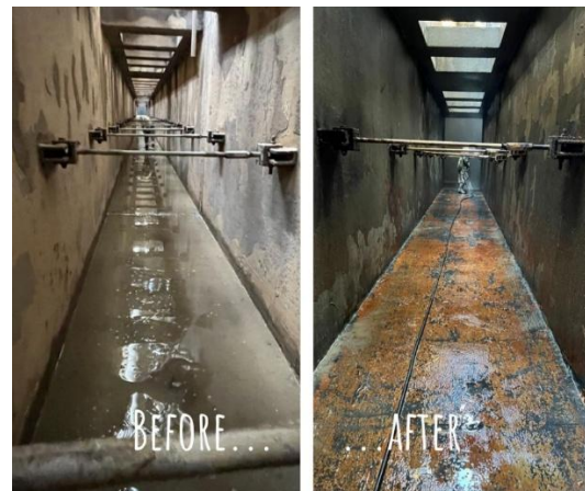
Figure 3 Cleared cooling tower channels (Source: Medway Cooling Towers Clean Ainsworth Civils and Engineering Limited AC&E )
