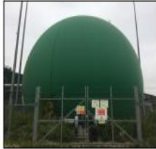
Figure 8: Double membrane gas bag.
