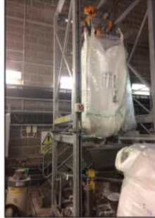
Figure 5: Polyelectrolyte hopper 2.
