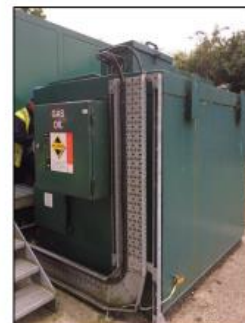
Figure 13: Diesel tank, next to inletworks.
