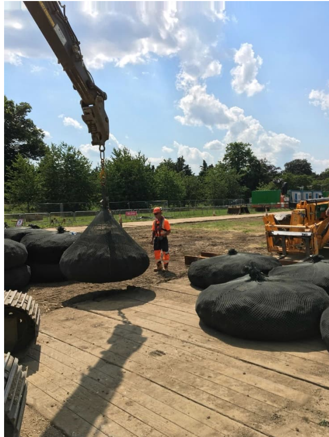
Figure 14. Rock filled bags being used at Black Potts Weir
