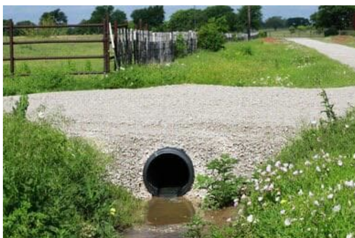
Figure 4. Piped ditch crossing example
