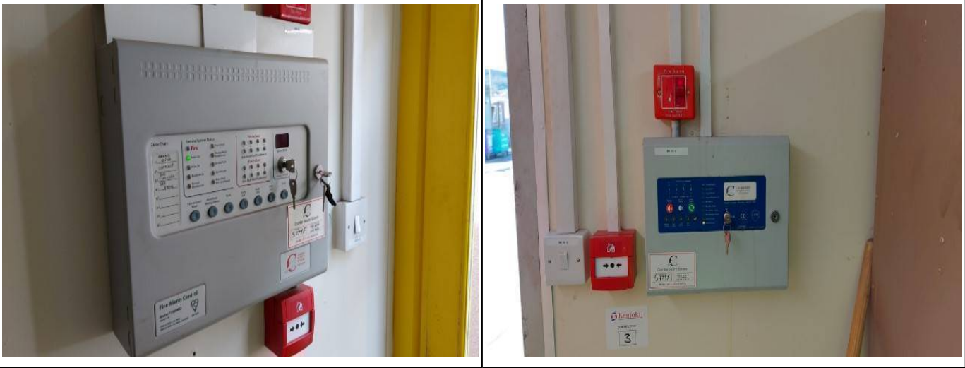
Description: Fire alarm panels.
