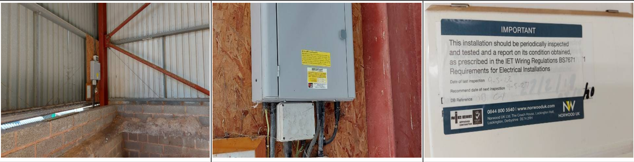
Description: Examples of electrical incoming and test labels.
