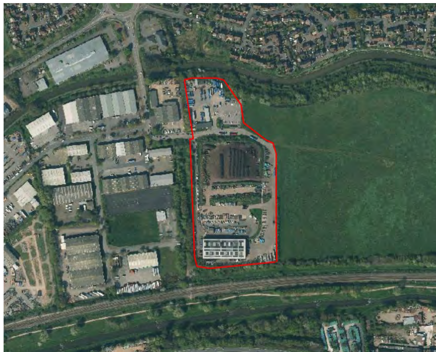
Plate 2: Aerial photograph with red line annotation indicating site boundary (Source: Ordnance Survey 100022861).
