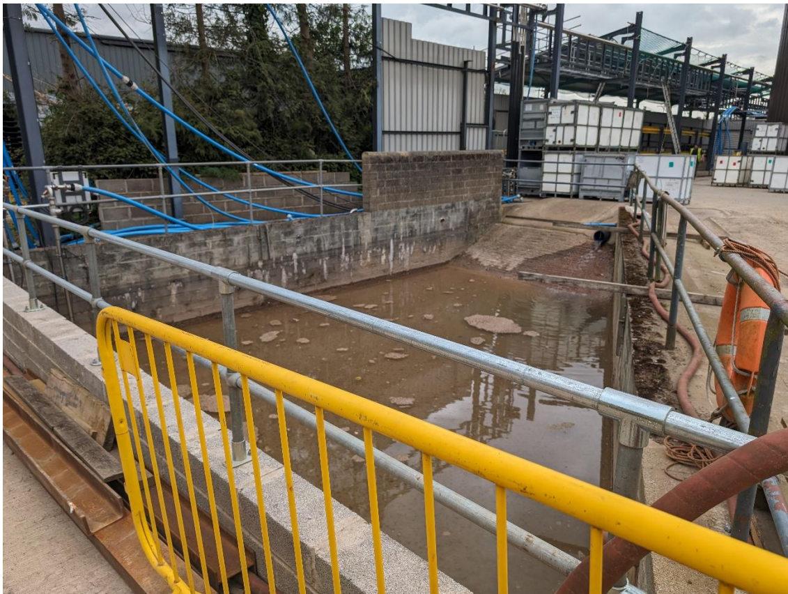
Photograph 12 –Yard run off storage and settlement pit
