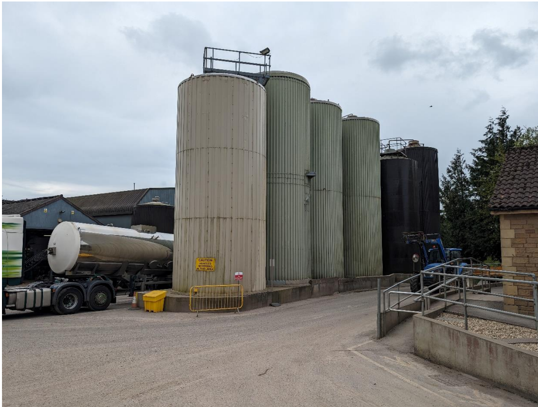
Photograph 18 –Looking south between main office and milk silos near site entrance
