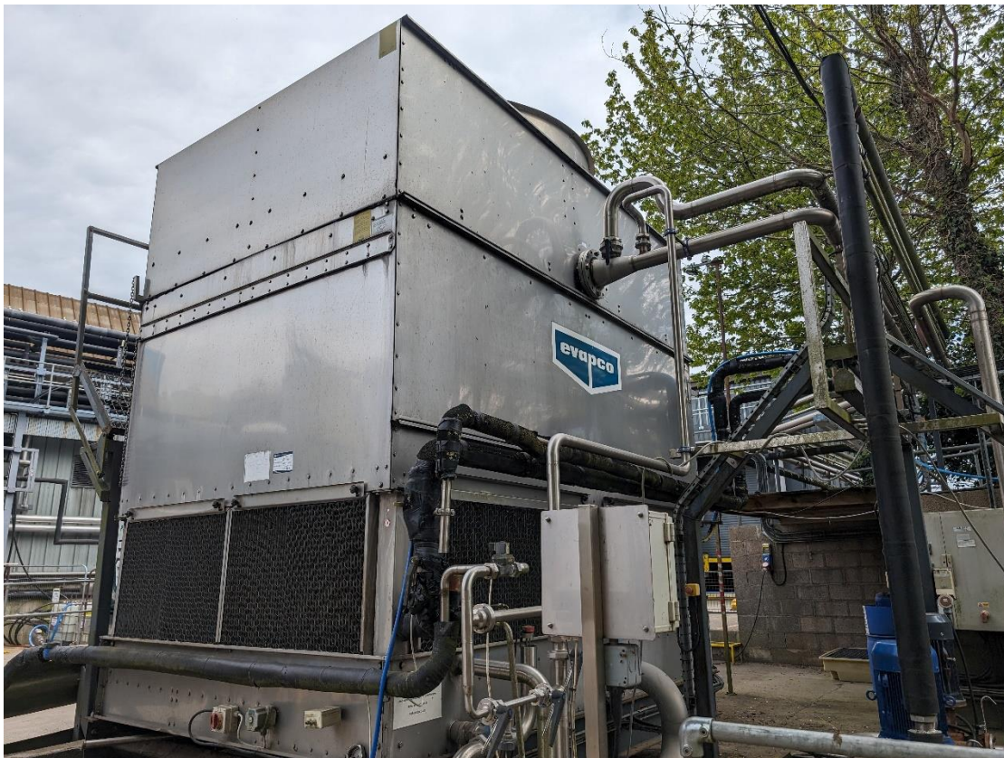
Photograph 25 – Cooling tower
