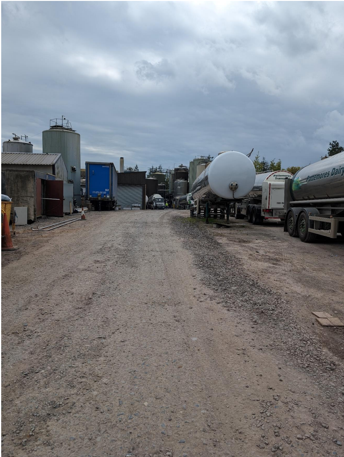
Photograph 19 – Looking south towards boilers 2 and 4
