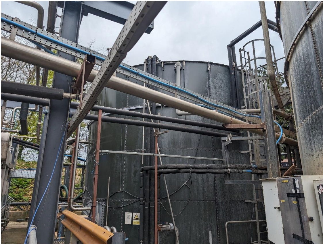
Photograph 6 – Balance tank with Effluent Treatment Plant Area
