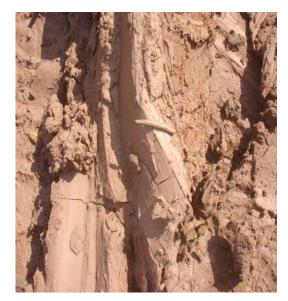
The basal lining system. 1 metre thick mineral engineered geological barrier for application area
