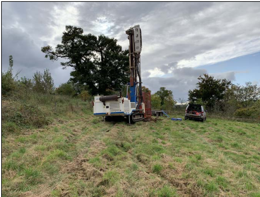
Figure 10: Soilmec SM-8G drilling and returns visible
