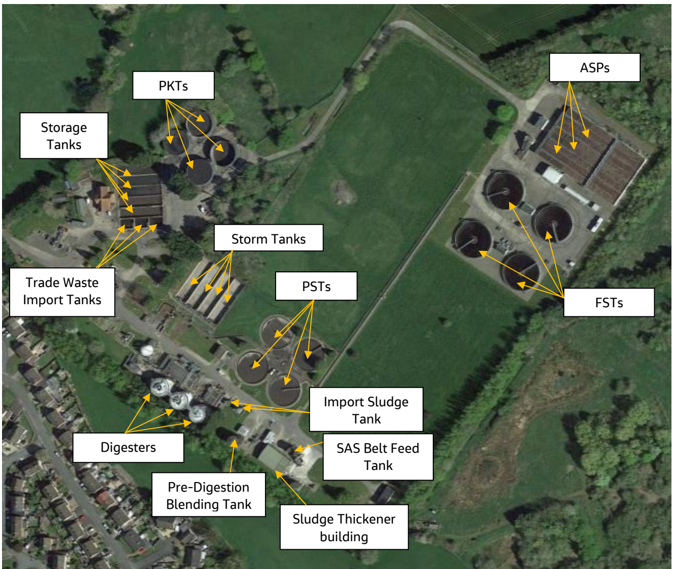
Figure 2.2 Labelled image of Monkmoor Sewage Treatment Works
