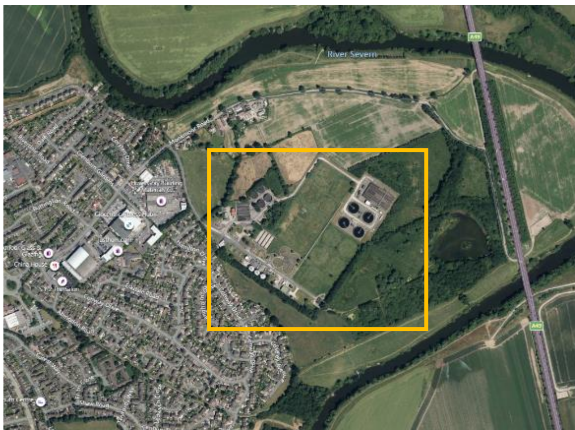
Figure i Satellite view of Monkmoor Sewage Treatment Works
