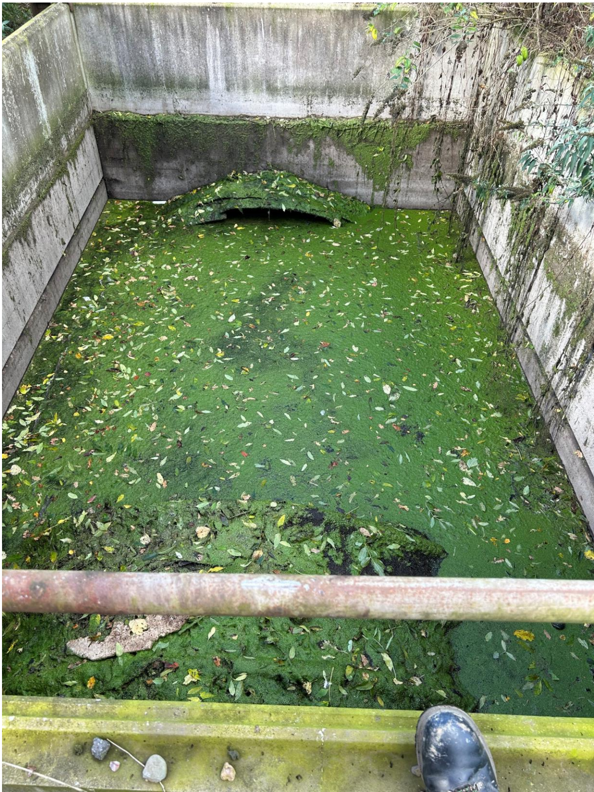
200,000l tank extending underground
