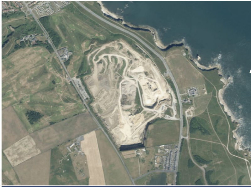
Image 1 – Immediate Site Surroundings
