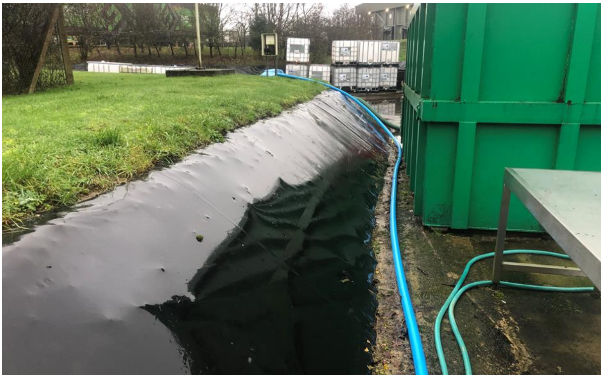
16. Secondary containment bund; North bund looking east
