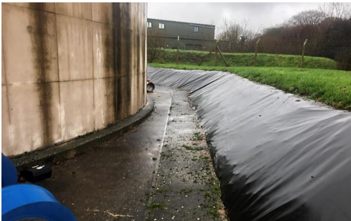
14. Secondary containment bund; South bund looking east
