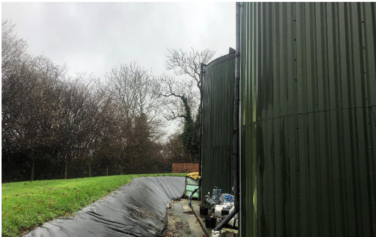
13. Secondary containment bund; South bund looking west
