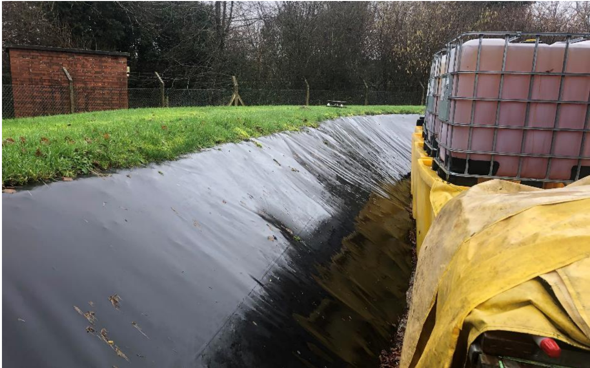
15. Secondary containment bund; South west corner bund looking west
