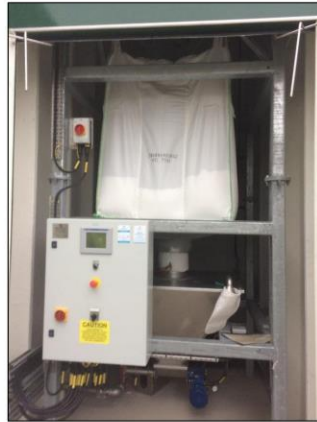
Figure 11: Polyelectrolyte dispenser 1.
