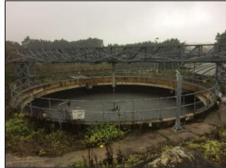
Figure 8: Post digester 1, open.
