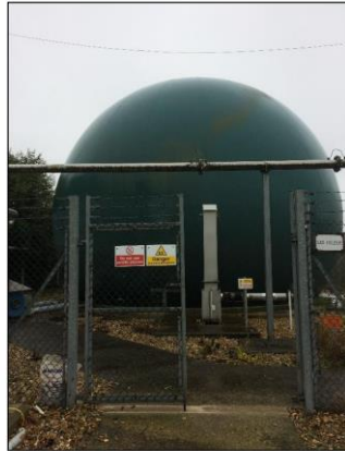
Figure 13: Double membrane gas bag.
