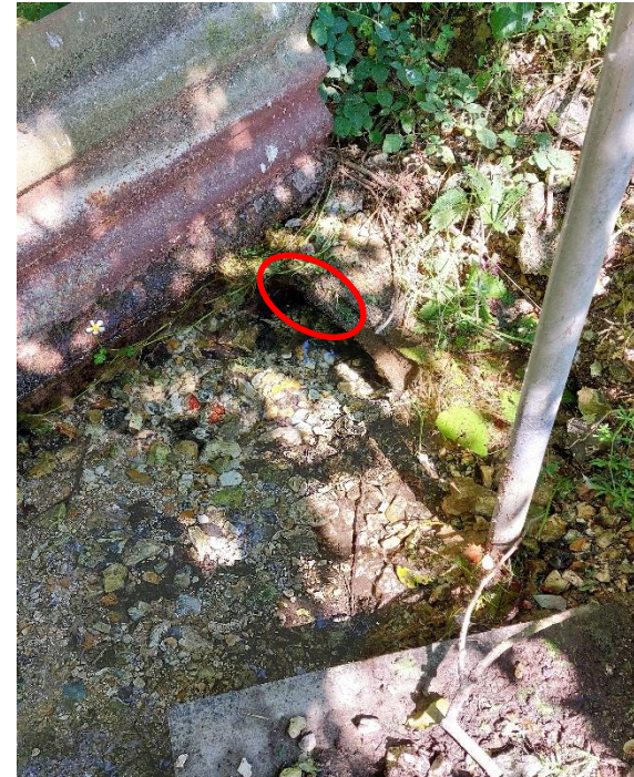
Outlet 2a: R block outlet
