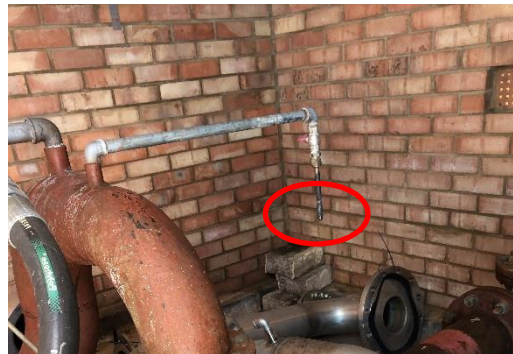
Inlet 4b: factory BH 2
