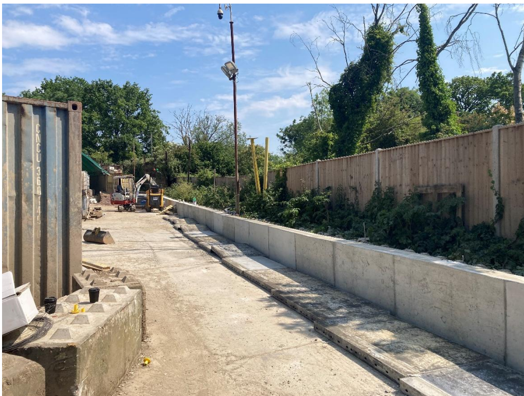
Image 10 – Tertiary Containment Wall during construction – LTP lower yard – View Towards D8a / Bunny Lane from D8b (Lowest point)
