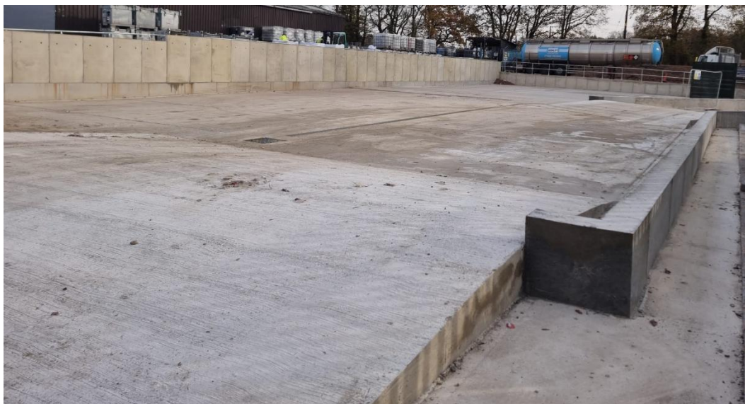
Image 12 - View from far side of roller bund in B towards bunny lane
