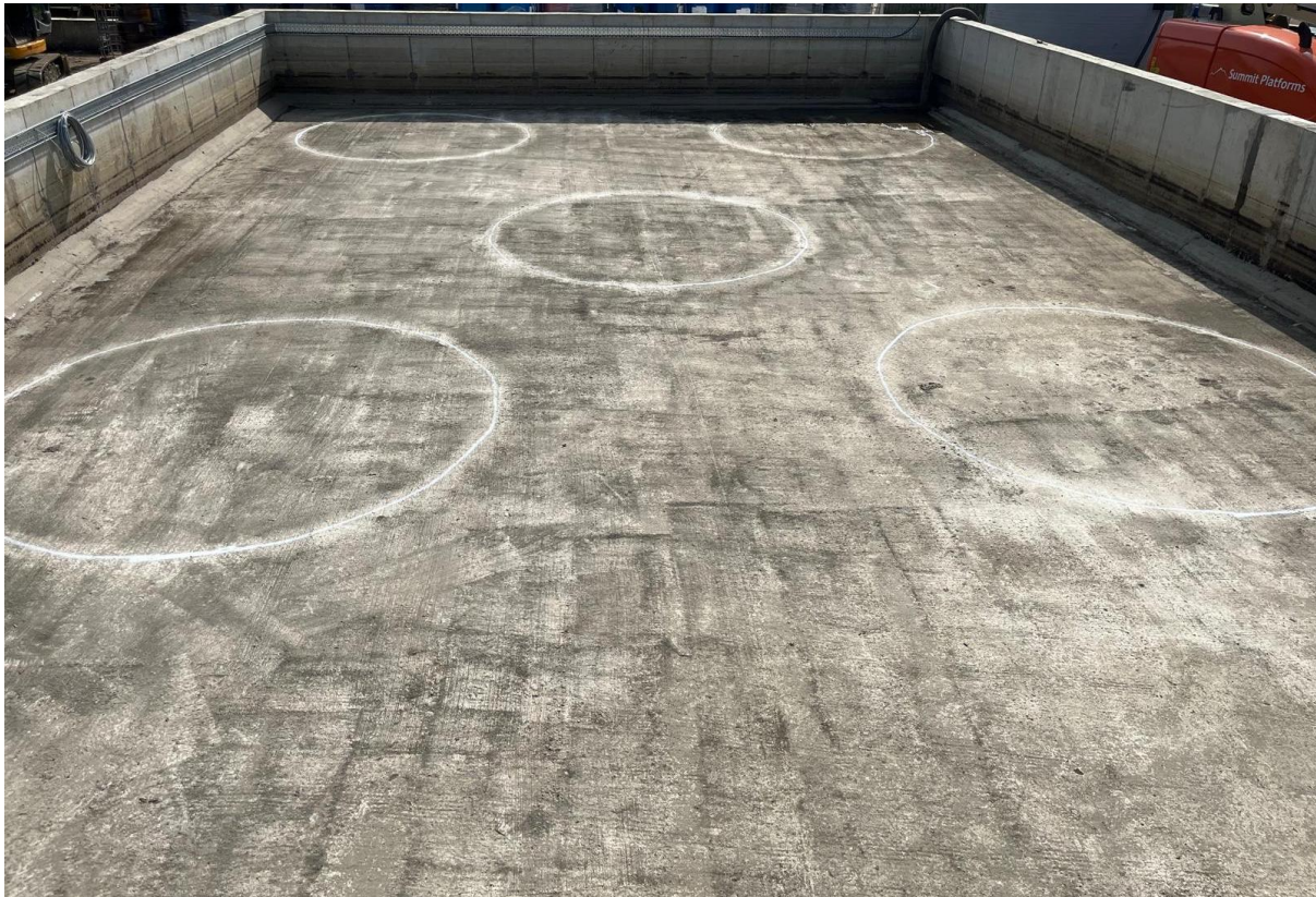
Image 7 – Tank Farm Bund prior to tank Installation
