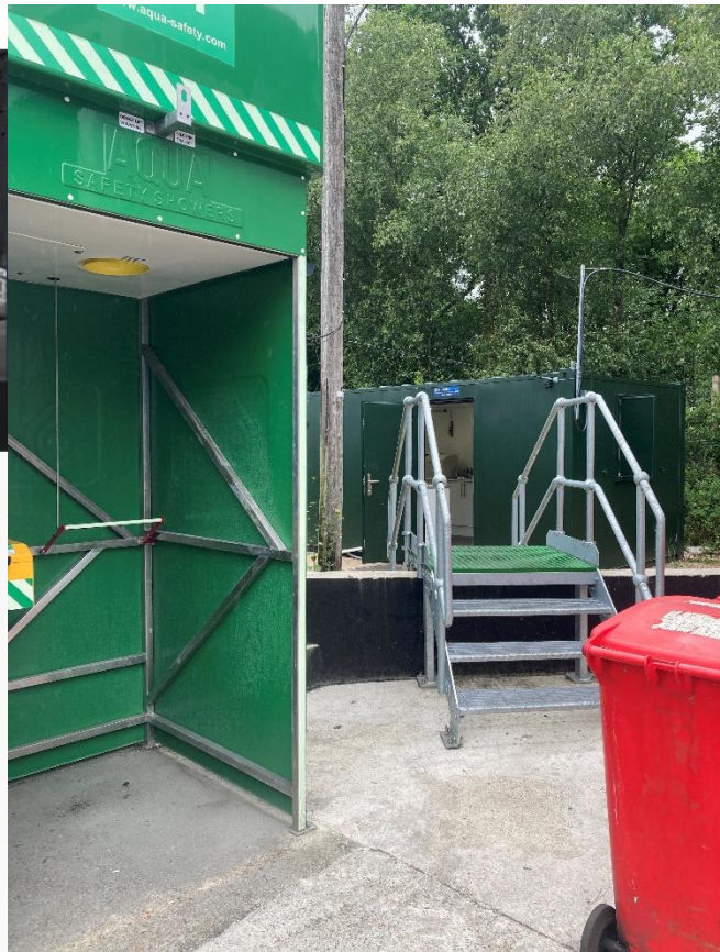
Image 19 – Tertiary containment wall adjacent to bay A2 & steps to onsite laboratory in background
