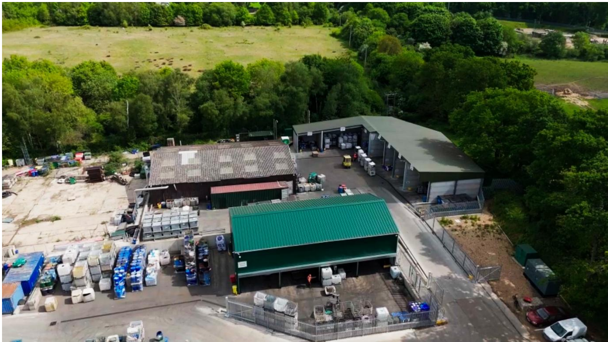
Image 14 - Aerial photo looking towards transfer station June 2025 during operations – Green building in foreground is plastics recycling building. Oliver Green building in top right of picture is new transfer station, Old asbestos cement sheet roof building in centre is original transfer station building
