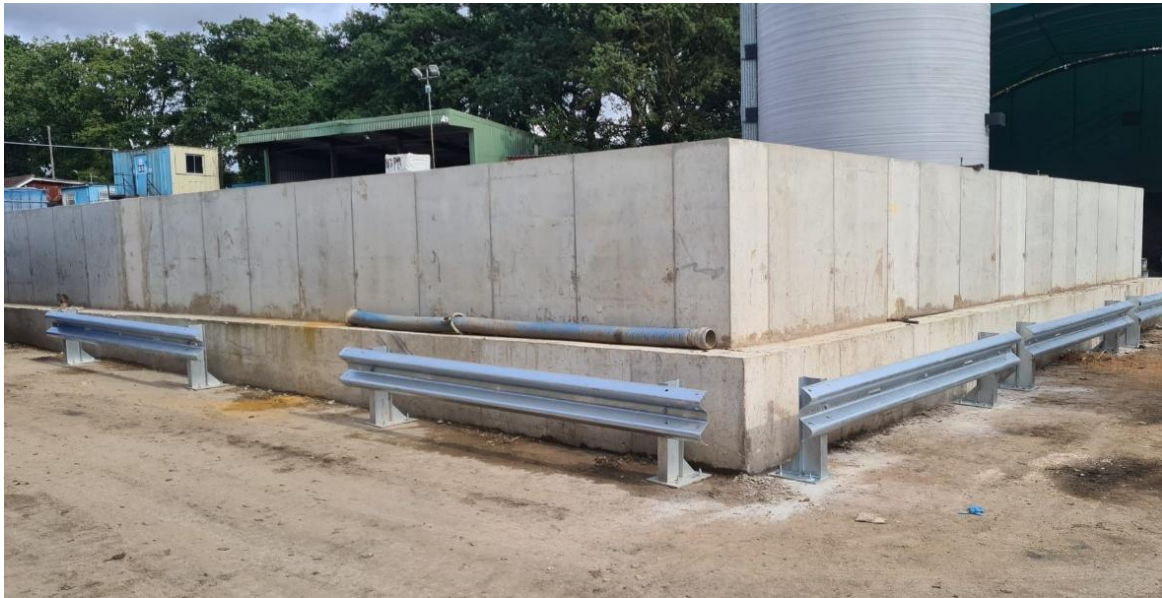
Image 8 – View towards offices from behind tank farm bund showing construction
