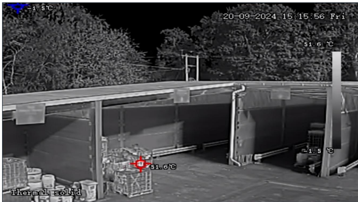
Image 15 – Thermal imaging camera view of half of new transfer station and offload area
