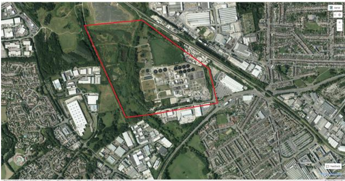
Figure 1: Satellite view of Swindon Sewage Treatment Works
