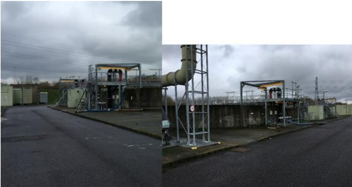
Inter-site Sludge Reception Points
