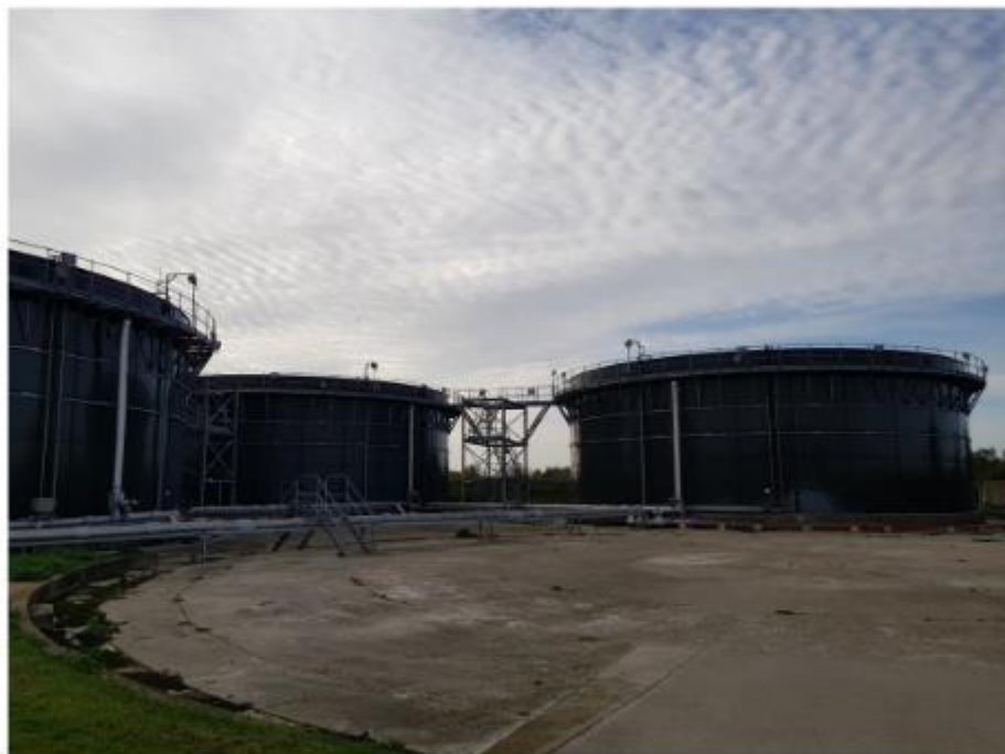
Photo of area of the three secondary digester tanks on site. Digested sludge is transferred to the digested sludge dewatering plant.
