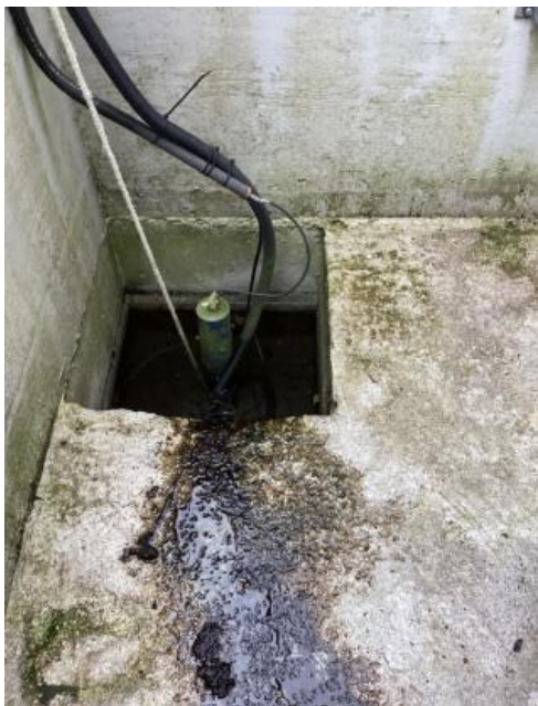
Photos 1 and 2 – Bund Before Photos
