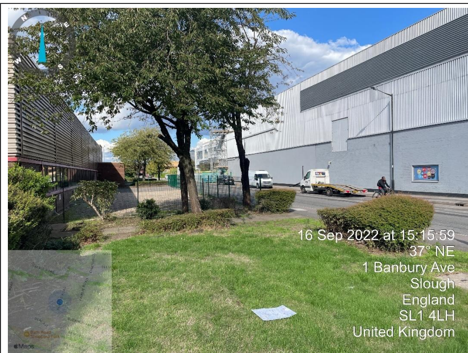
40. View north along the eastern site boundary with Dundee Road
