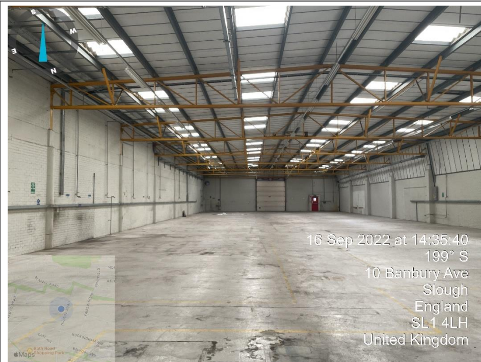
25. View of the inside of the Bay 11 warehouse
