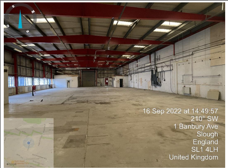
28. View of the inside of the Bay 13 warehouse
