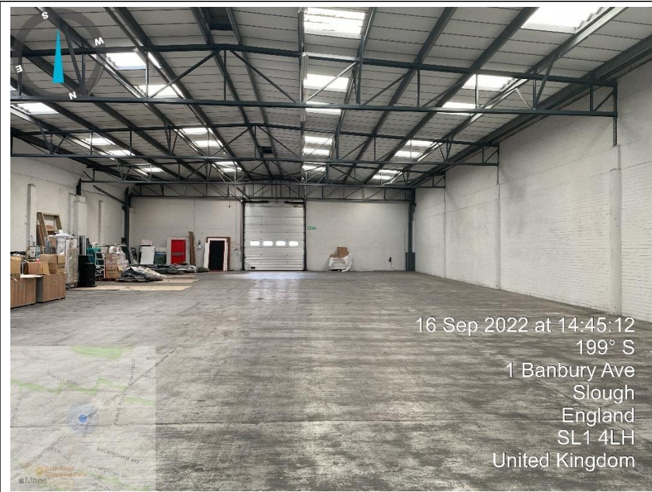
27. View of the inside of the Bay 12 warehouse
