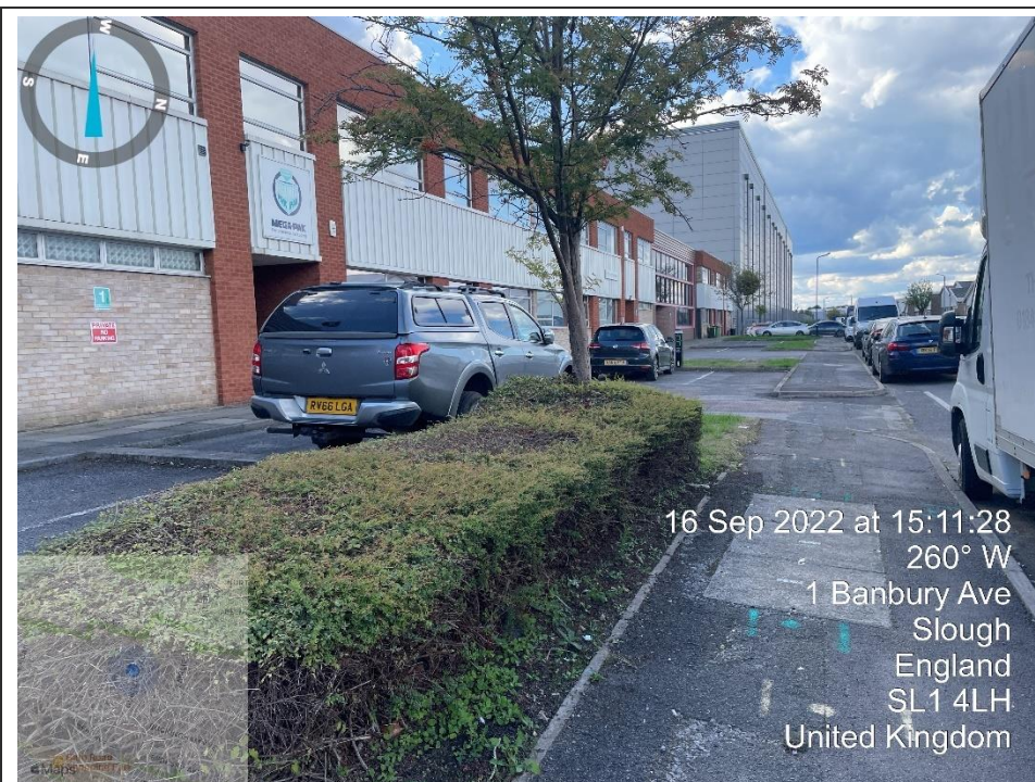
36. View west along the northern site boundary with Banbury Avenue showing the front of the building, soft landscaping and car parking areas
