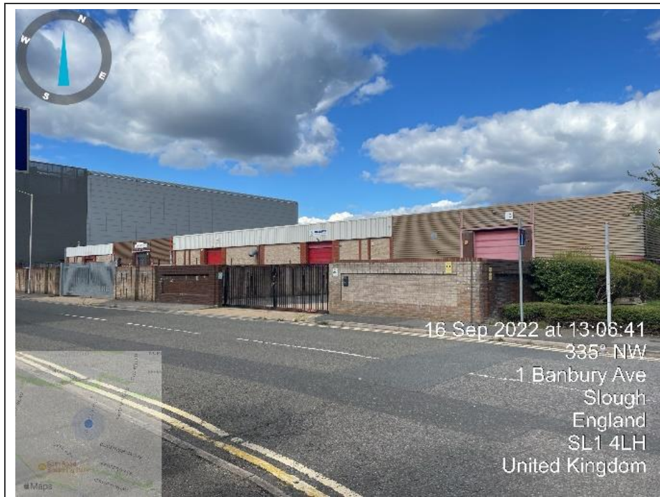
1. View northwest of the rear of the site from Oxford Avenue
