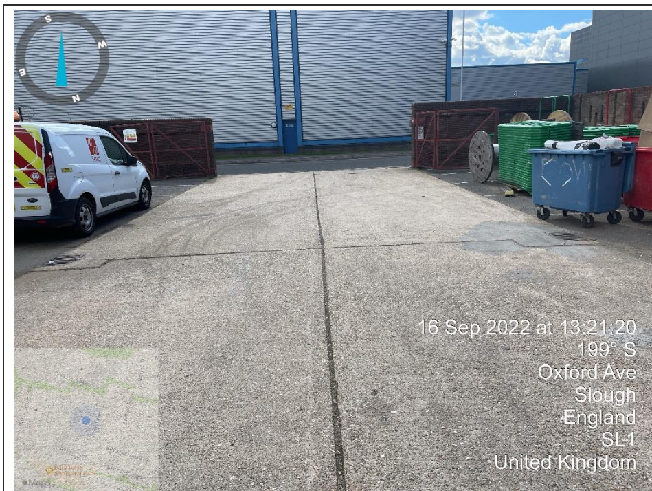
9. View south of the rear loading bay/ vehicle parking area of Bay 10
