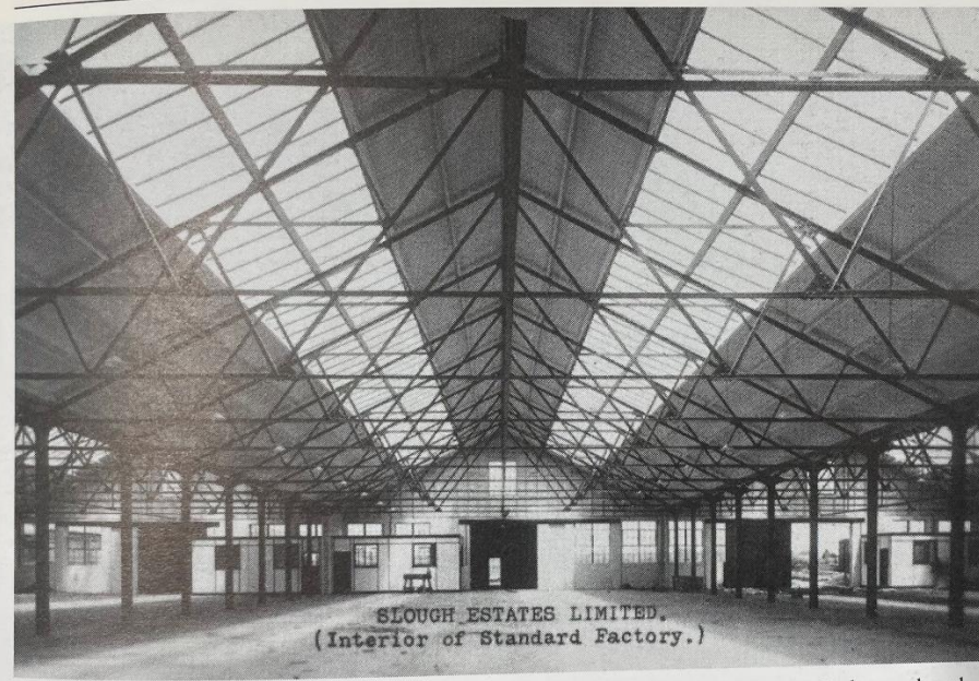
Photo of the inside of a typical factory unit from the 1920s and 1930s
