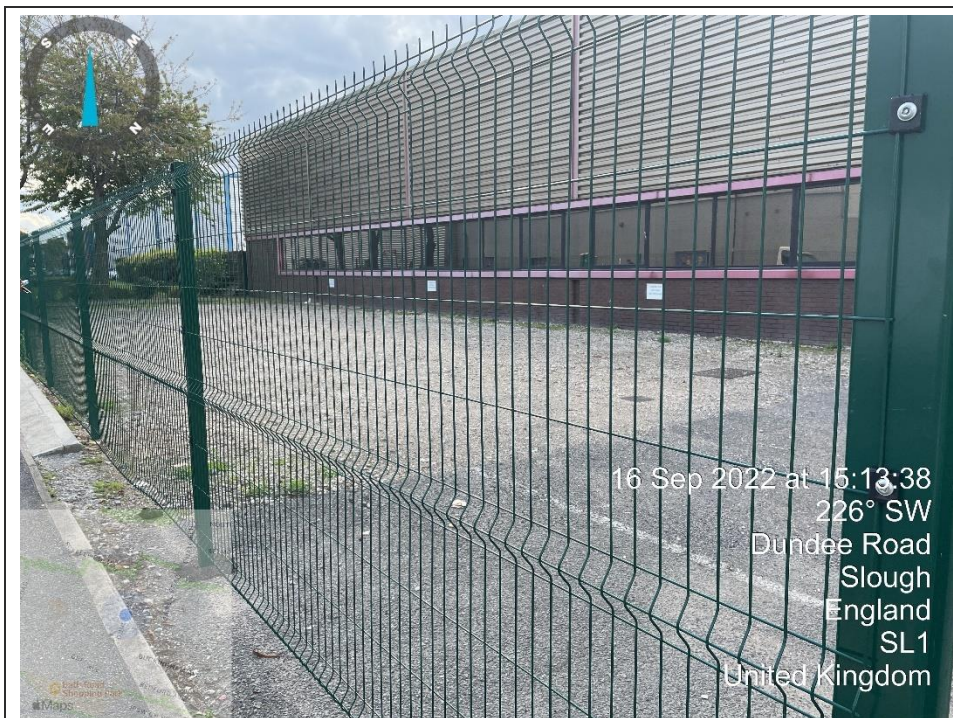
39. View southwest from the eastern site boundary of the gravel car park area to the east of Bay 13
