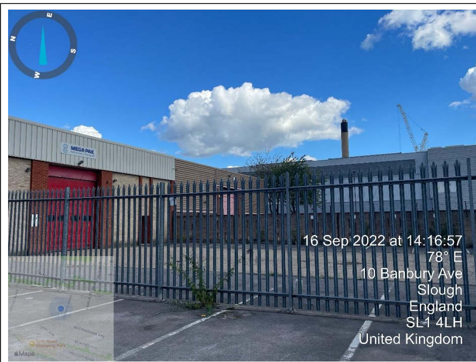
24. View east of the rear loading bay/ vehicle parking area of Bay 12, formerly occupied by Mega Pak
