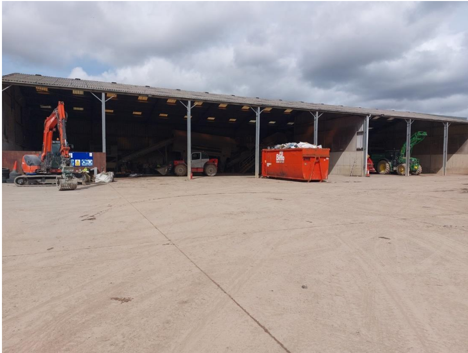
Plate 1. View of front of Transfer Station Shed
