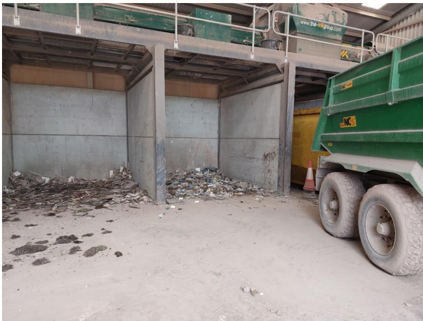
Plate 4. Showing Construction of storage bays beneath picking station
