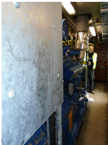
Photograph 13- CHP Container Interior
