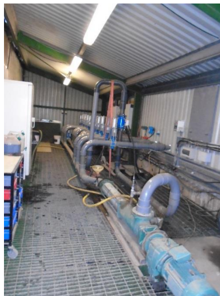
Photograph 4 – Flow meters used to transport the food waste to the digesters.
