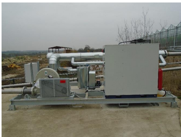
Photograph 13- CHP Container Interior
