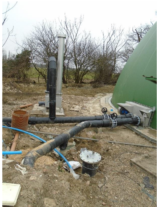
Photograph 16 – Overpressure valve
