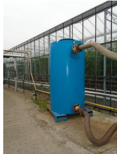
Photograph 8 – Water Trap
