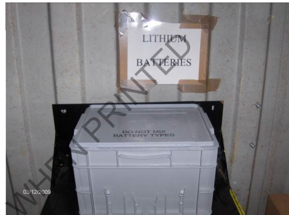
Battery box (0.1 m 3 ) storing lithium batteries in a dry environment.
