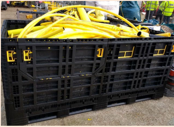
Double magnum can only be used to store PE pipe. (volumes typically 250kg).
