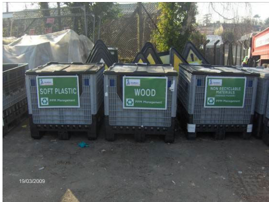
Back loading for 3 waste streams (individual magnum capacity is approximately 0.8 m 3 ).
