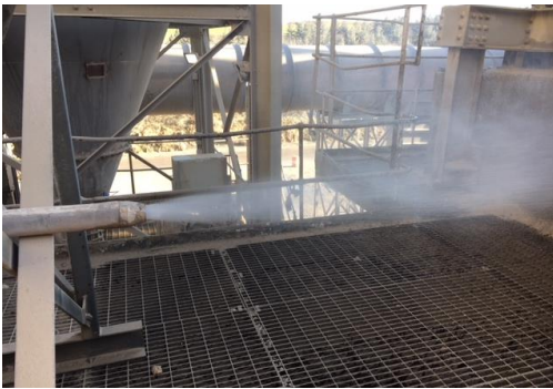
Water being atomised with compressed air
