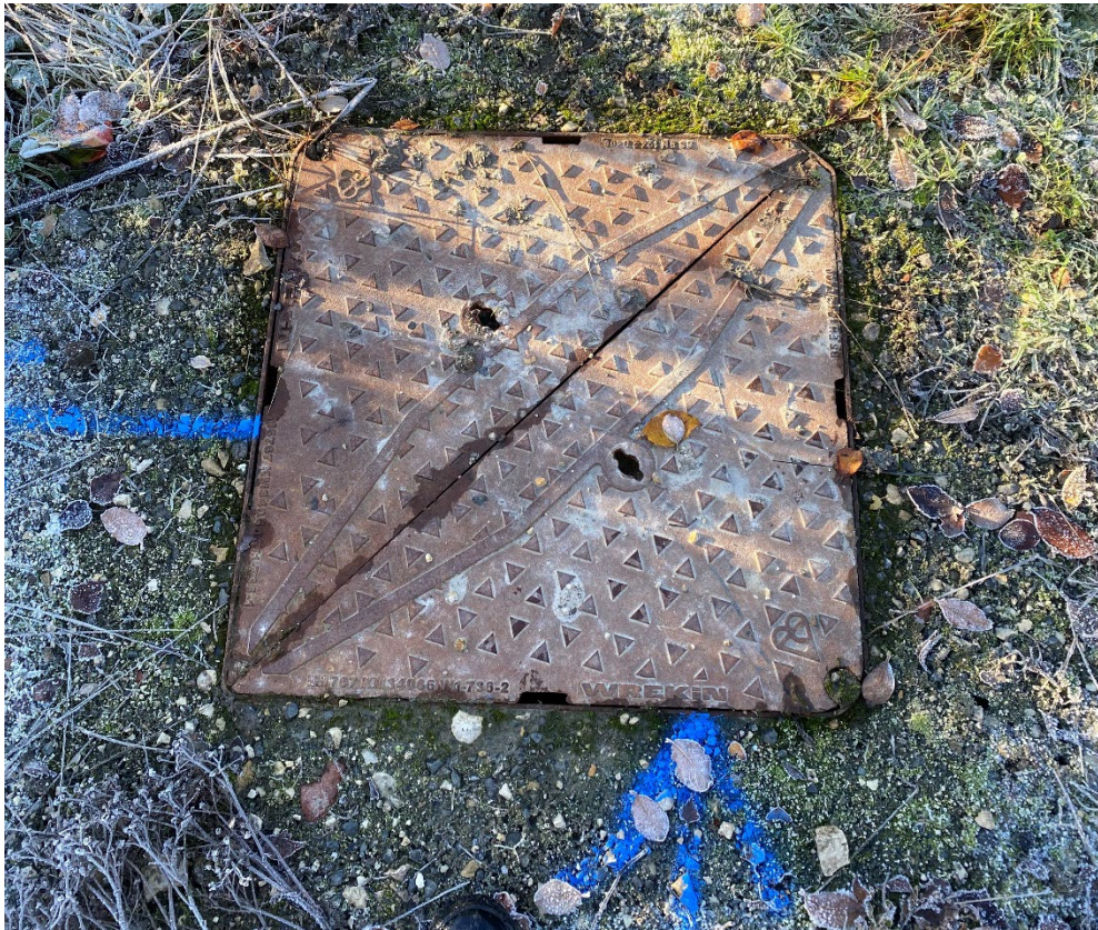
Photograph 7: Existing drain on site
