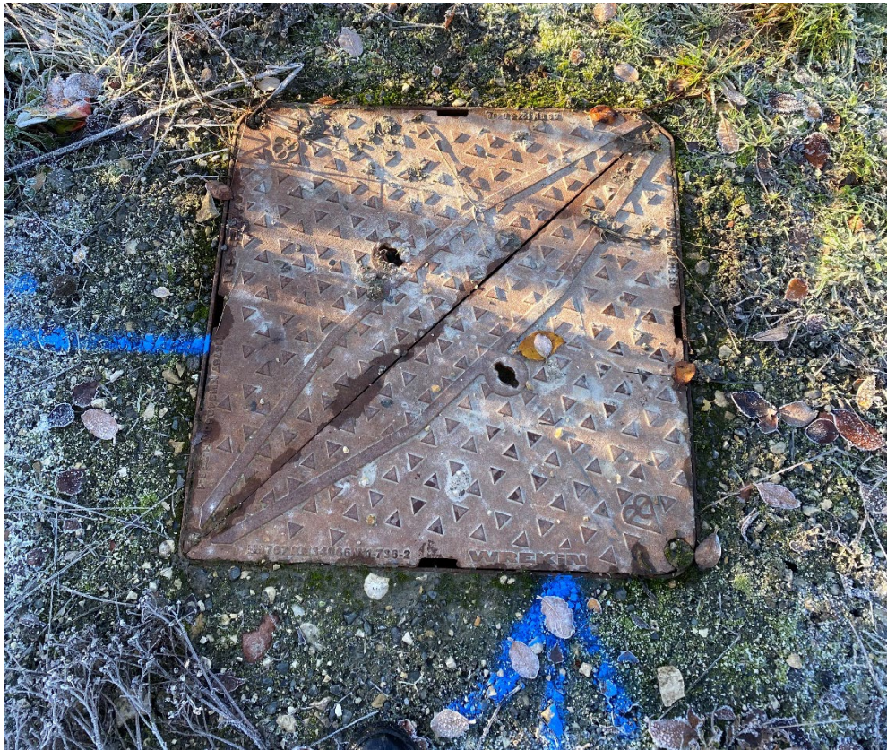
Photograph 7: Existing drain on site
