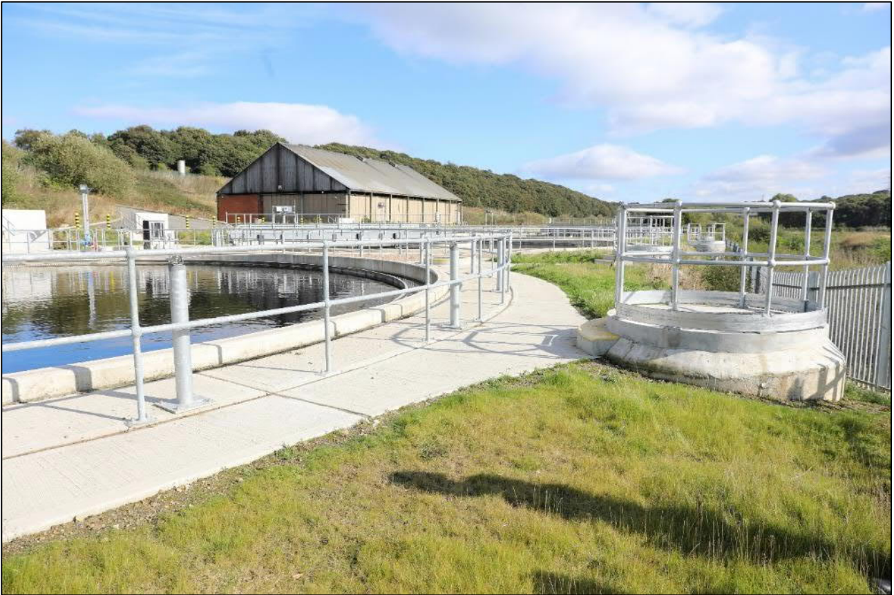
Figure 29. Sloping embankment south of the FSTs adjacent to sensitive receptor.
