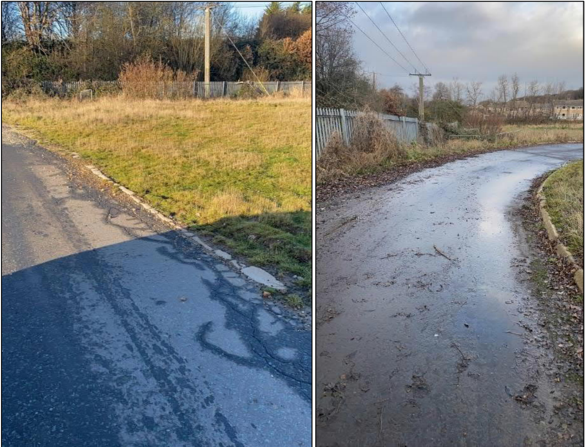
Figure 23 a) elevated bank with rough vegetation, b) curving access road with camber towards kerbed inner section.
