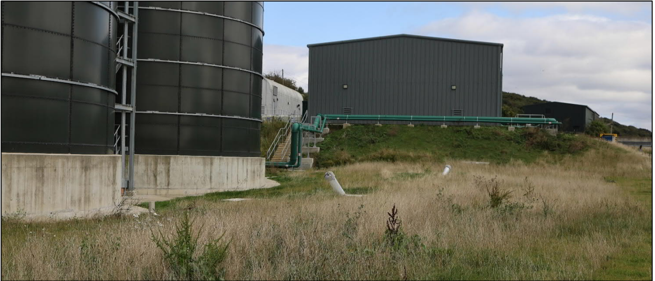
Figure 39 - Land rises to east of thickener feed tanks
