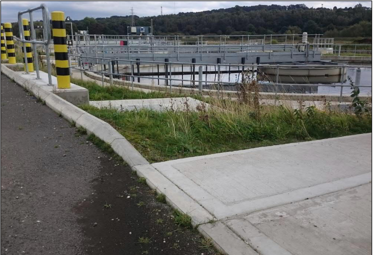
Figure 27. Section of dropped kerb on access road near FSTs.
