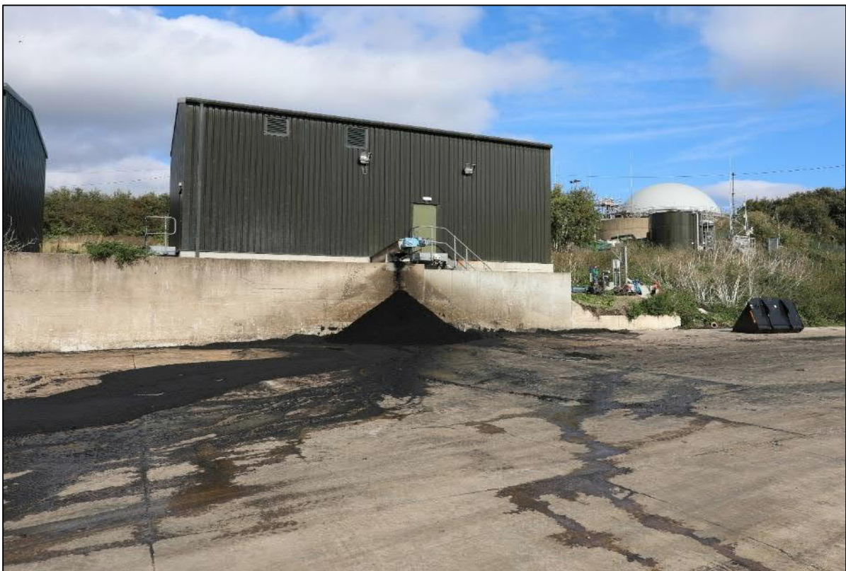
Figure 15. Sludge cake conveyor and pad.
