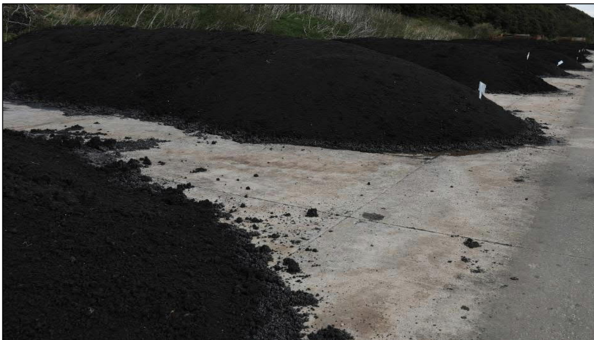
Figure 16. Sludge cake storage pad.
