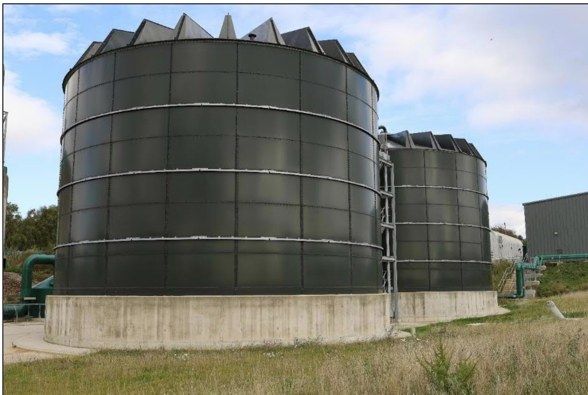
Figure 10. Drum thickener feed tanks (2 no.).
