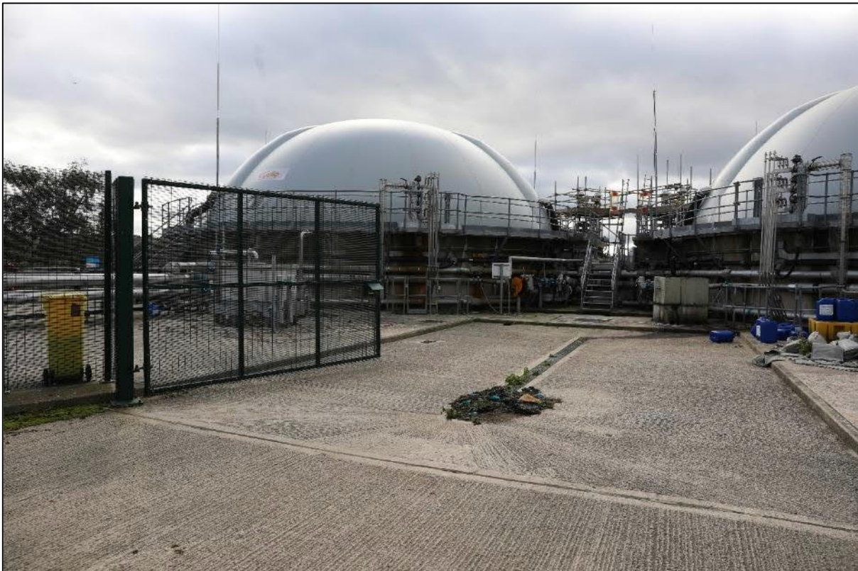
Figure 12. Digesters (2 no.).
