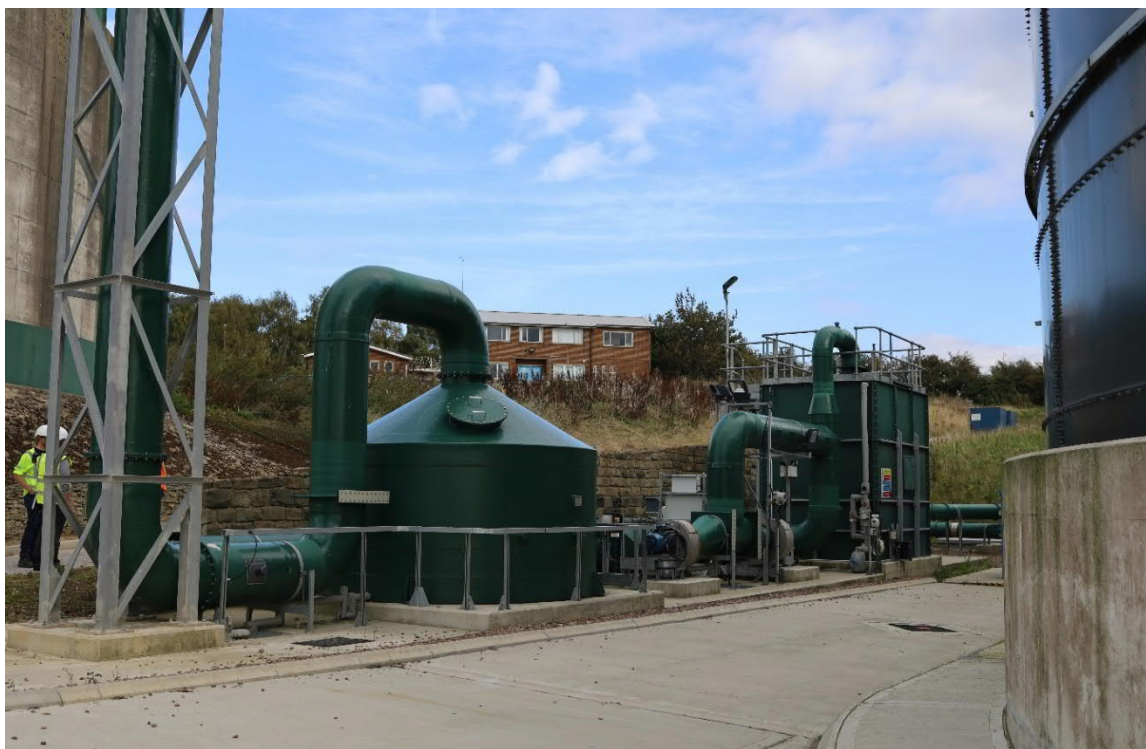
Figure G Odour control unit
