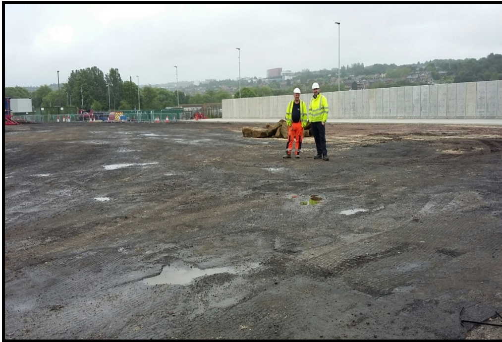
Photograph 41 Looking south-west across the Waste Transfer and Treatment Area showing the construction of the concrete bunkers to the west. It is proposed to return these concrete bunkers across the south end of the site to form the quarantine and fire water holding areas. The concourse area above will be surfaced with an impermeable bituminous binder and surfacing materials.
