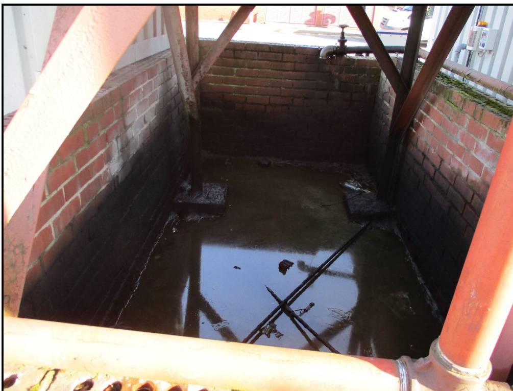
Photograph 7 Bunded area below diesel tank shown in Photograph 5 showing some deterioration and requires emptying of water and fuel residue (located outside the proposed permit boundary)
