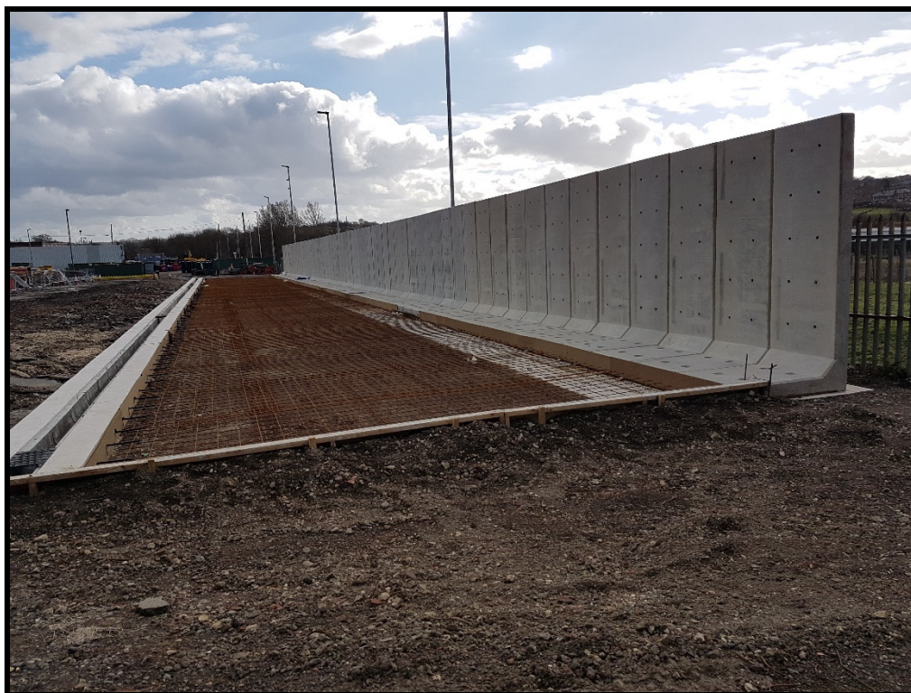
Photograph 39 Commencement of construction of waste bays along western boundary of Waste Transfer and Treatment area. Fall towards Birco strip drain apparent (facing south)
