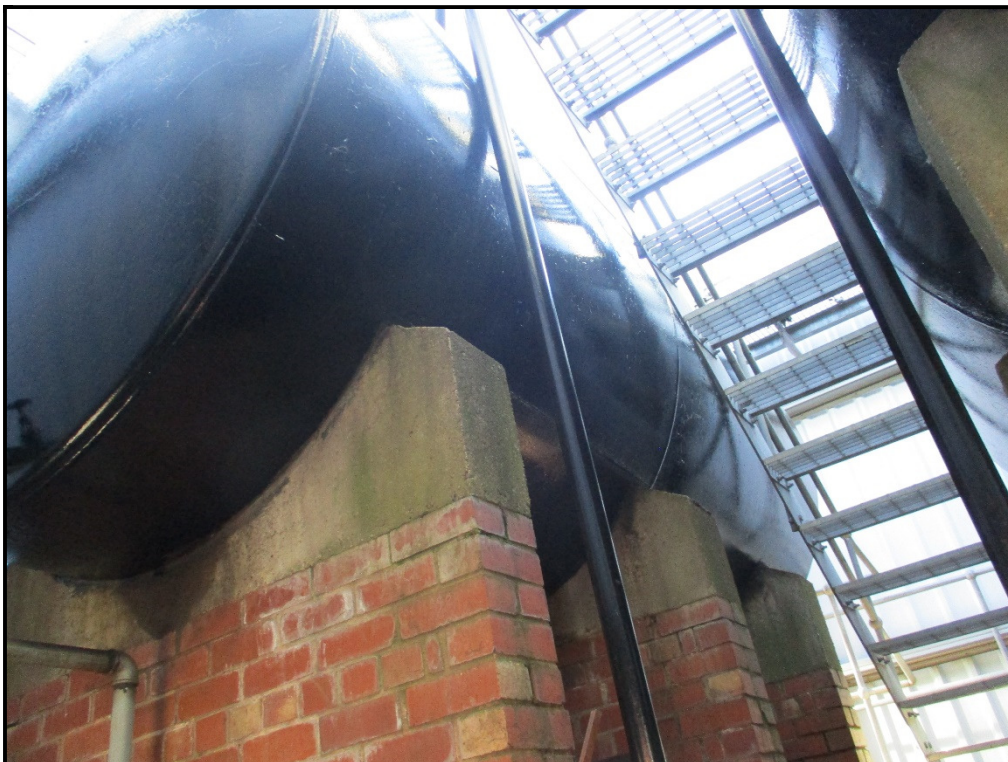
Photograph 2 View of fuel tanks within the bunded area shown in Photograph 1 (located outside the proposed permit boundary)
