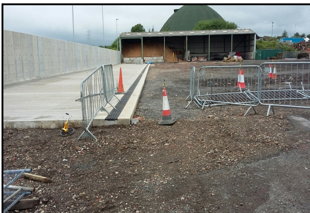
Photograph 40 Looking north across Waste Transfer and Treatment Area following completion of the base of the concrete bays (location of MH1/MH4 and fire water holding area in the foreground).
