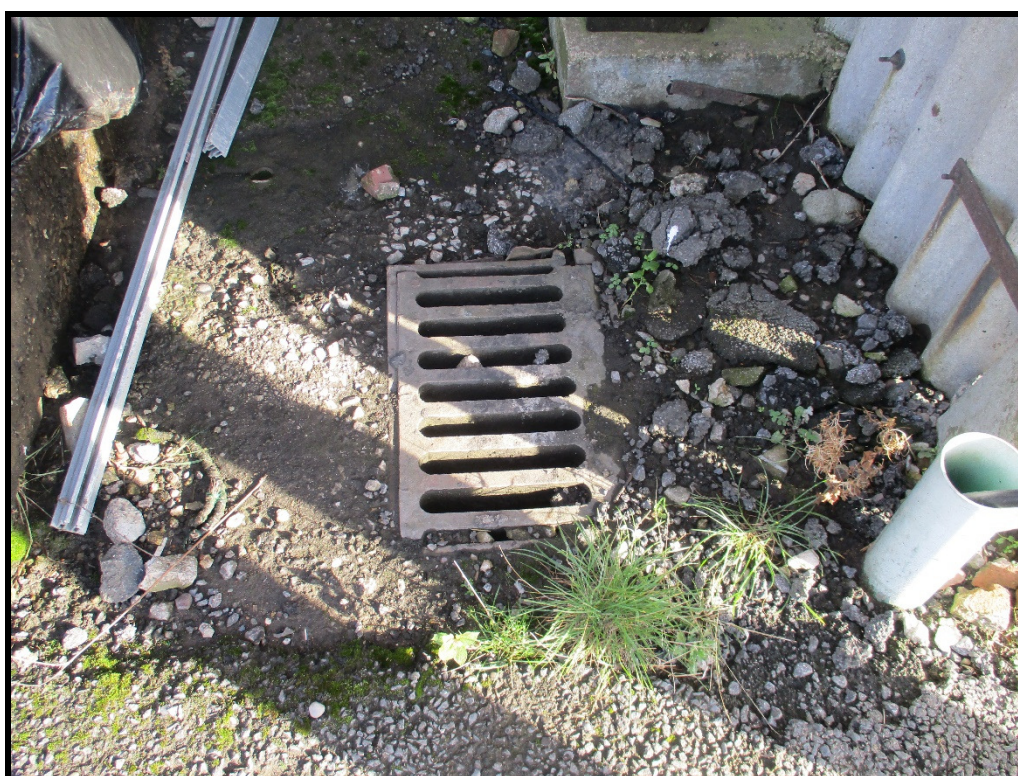
Photograph 32 Open surface water drain located between the water storage tank (Photograph 20) and the adjacent shed to the south
