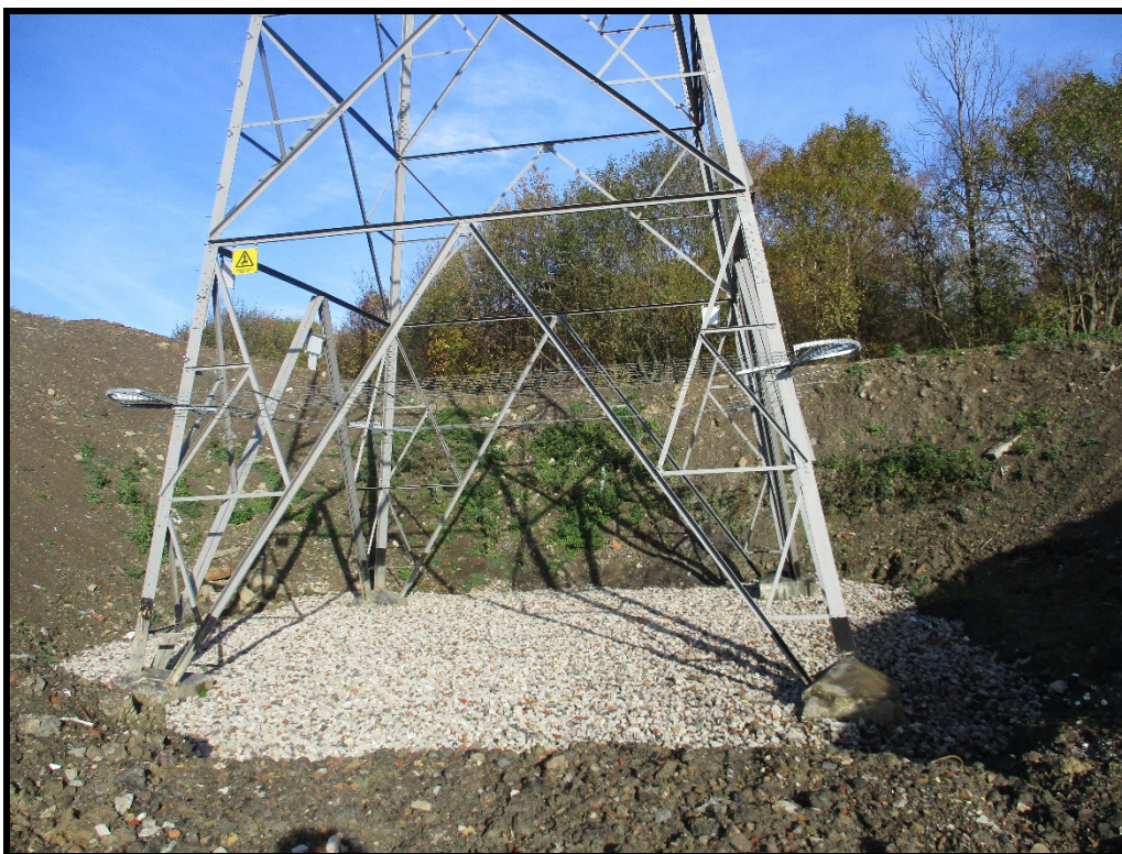
Photograph 29 Upper part of the proposed site showing pylon base surrounded by a protective soil bund adjacent to the green waste storage and bulking area
