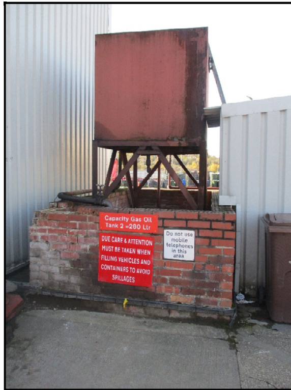
Photograph 5 Diesel tank with brick bunded containment, showing some external deterioration (located outside the proposed permit boundary)
