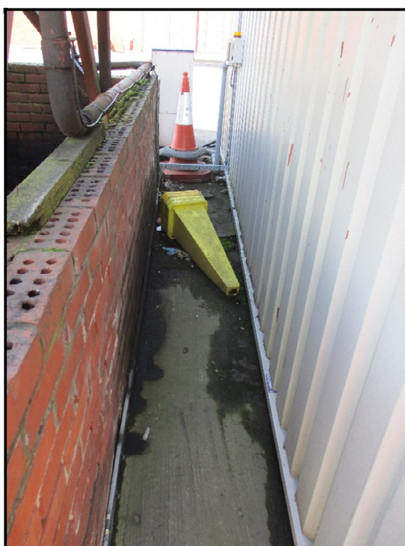
Photograph 8 Evidence of fuel / water seepage from the bunded fuel tanks area (located outside the proposed permit boundary)
