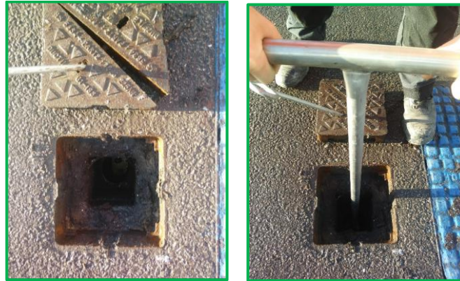
Figure 14: Example penstock valve which will be installed in the surface drainage system
