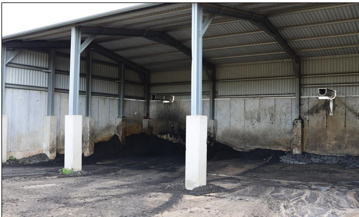
Figure 16. Sludge cake barn.
