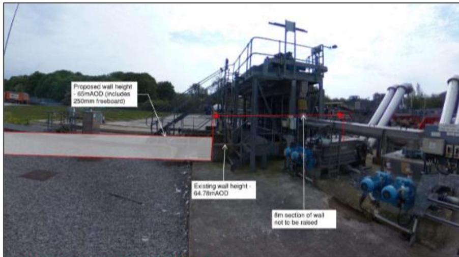
Figure 4 Inlet works section to exclude freeboard
