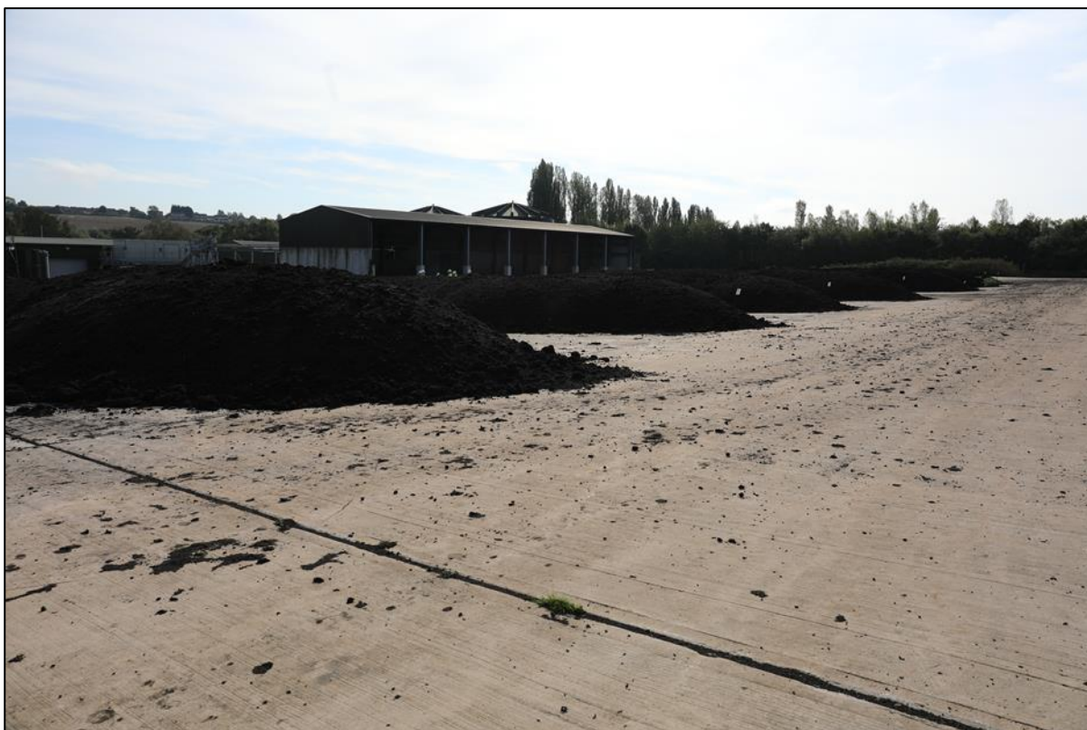
Figure 17. Sludge cake storage pad.
