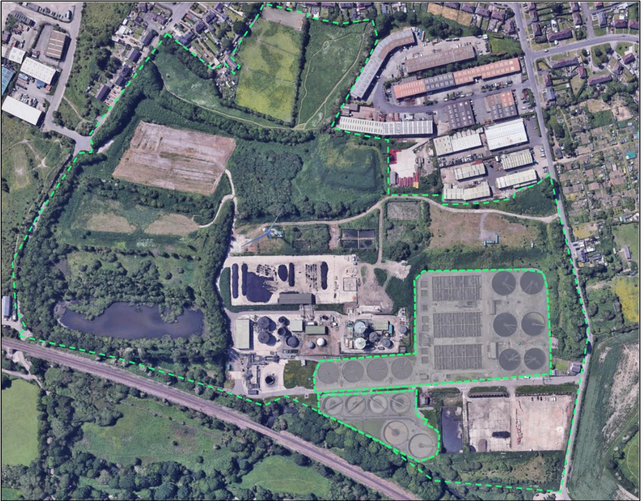
Figure 1. Old Whittington STF aerial view. Permit boundary in green. © Google, 2021
