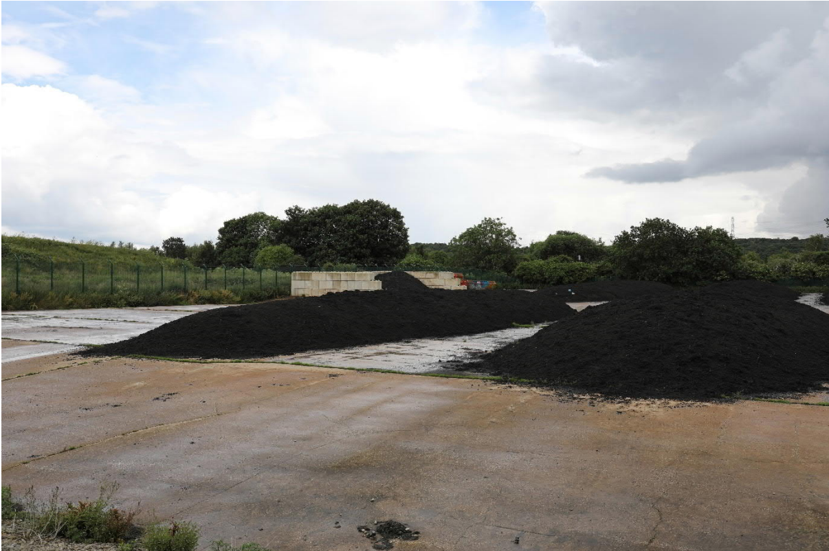
Figure 16. Sludge cake storage pad.
