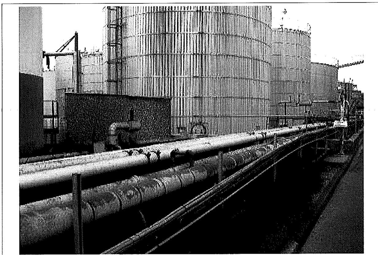
PLATE 2: Area 3 pipelines; extensive staining on gravel surfaced is evident on the ground beneath the pipes
