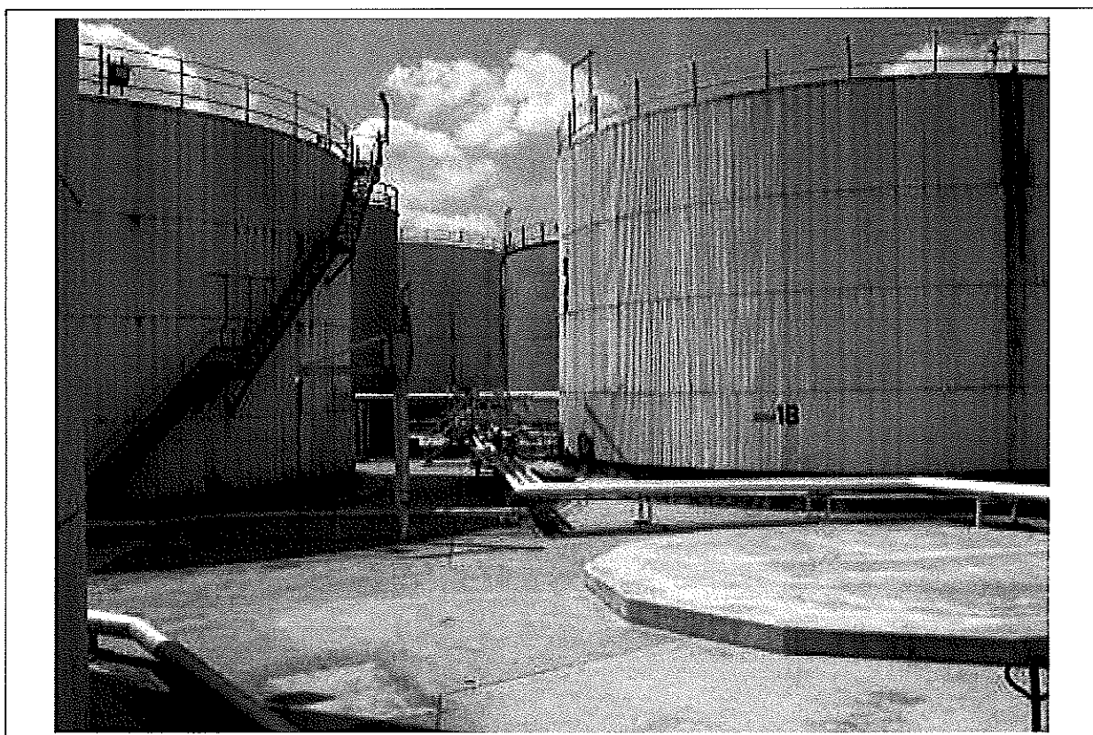
PLATE 4: Bunded ASTs in Area 3 (new)
