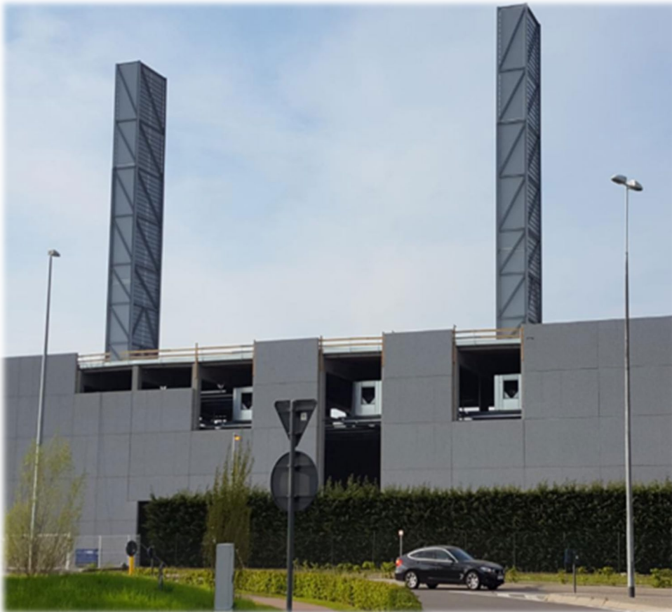
2x 50 m freestanding steelstructures with stainless steel flues made from sandwich panels.
