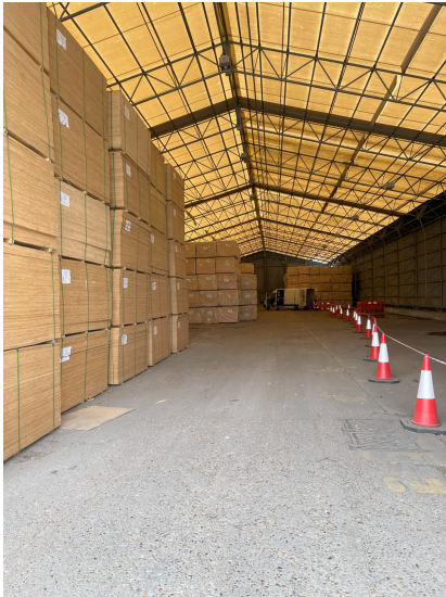
Photograph 9: Inside RUBB Building 36A
