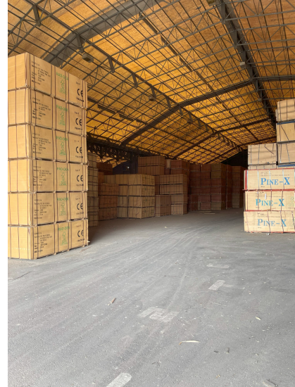
Photograph 10: Inside Building 3A
