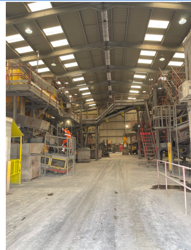
Photograph 6: IBA Processing Facility
