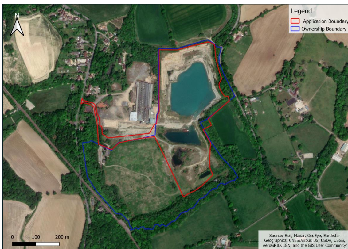
Figure 2-1 Aerial Imagery of the Site
